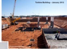
Turbine Building Prep
