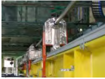
CRD shaft supports (view from above)
