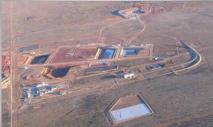
Aerial Photo Taken January 2012 by WCS Oblique photograph was taken looking to the north, with Stateline Road along the west (left) & Hwy 176 in the foreground (right), encompassing all the facilities at the WCS site in Andrews County Texas
