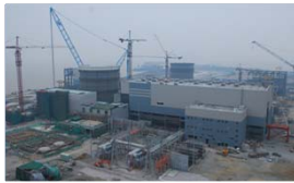
Sanmen site photo.
