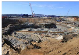
V.C. Summer site preparation.
