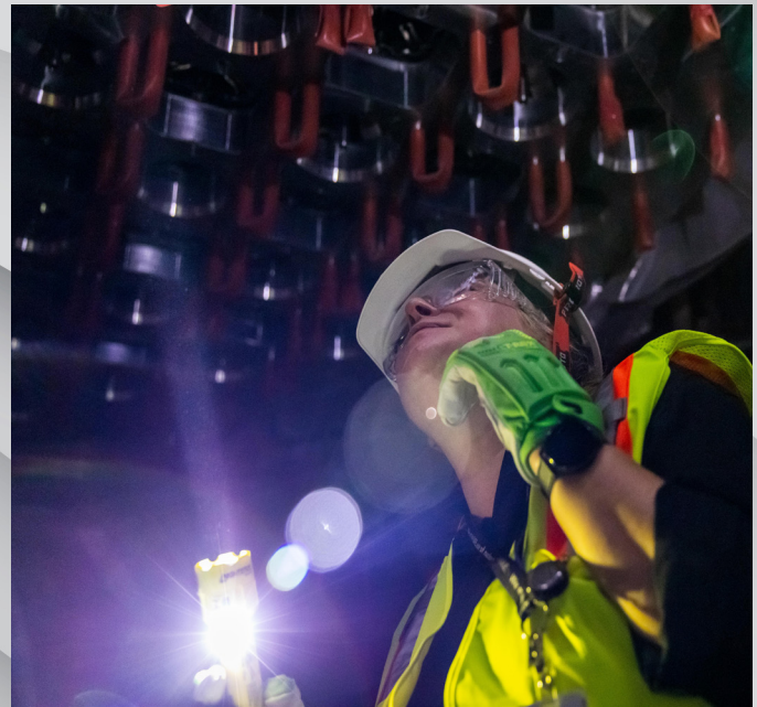
NRC Office of Nuclear Security and Incident Response Director Mirela Gavrilas observes new construction activities at Vogtle Units 3 and 4, in Georgia.
