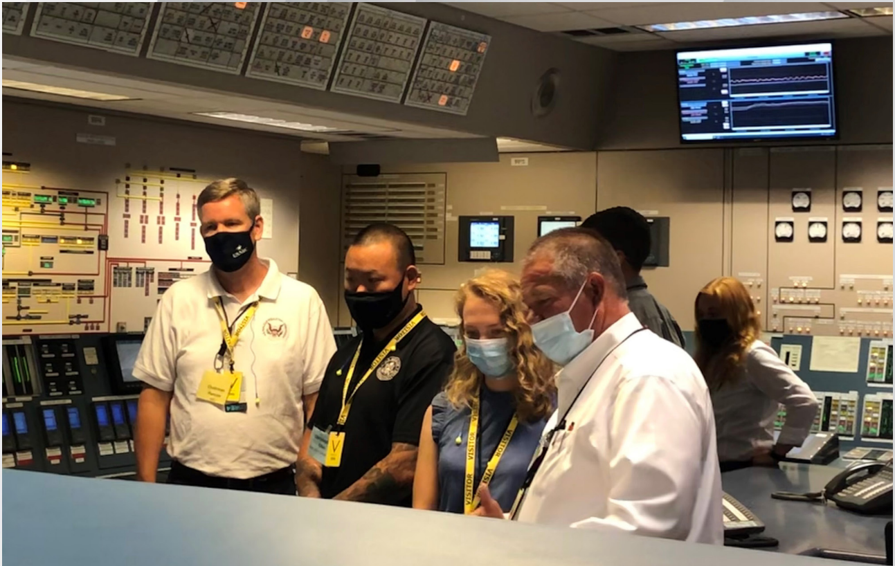
Chairman Christopher T. Hanson (left) observes plant operations, including a stop in the control room during his visit to the Salem and Hope Creek nuclear power plants in New Jersey.
