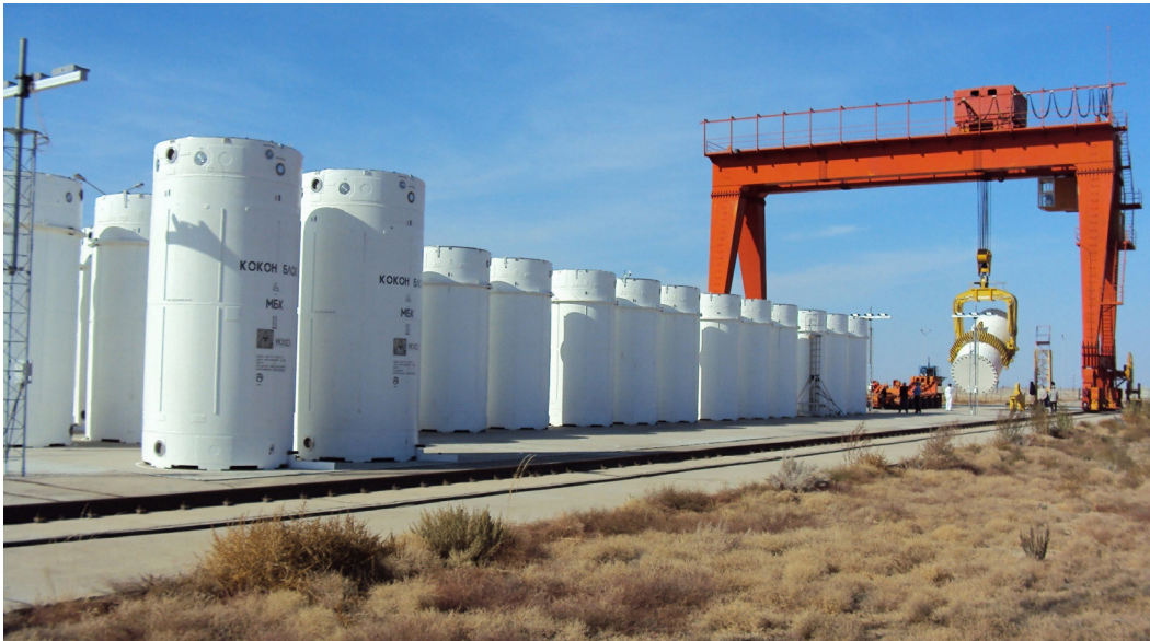
Massive containers hold spent nuclear fuel at safe and secure dry storage facilities. This photo shows, at right, dry cask recently loaded with spent fuel being lifted from a horizontal transporter to be placed vertically on a specially-designed storage pad. Courtesy of Sandia National Laboratories.
