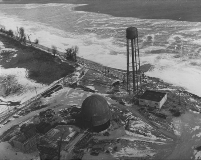
PRDC reactor under construction, 1958.
