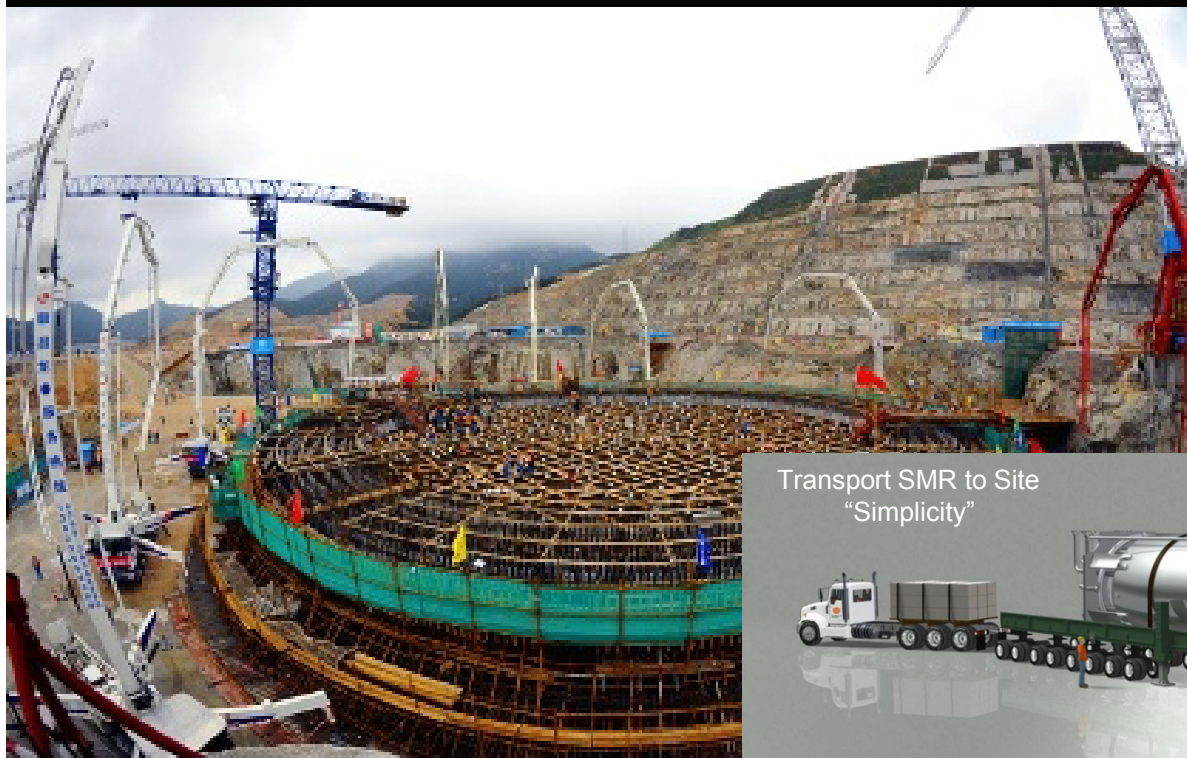
On-site Construction – “Complexity”
