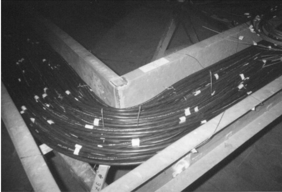
**Figure 4-3. Cable arrangement near corner of tray.**
