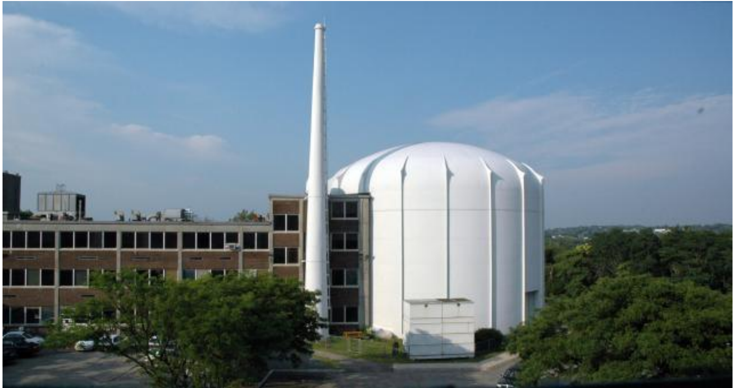
Research Reactor Building and Vent Stack
