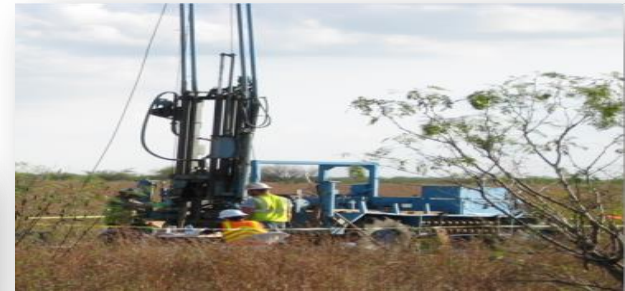
Bore hole drilling at Clinch River
