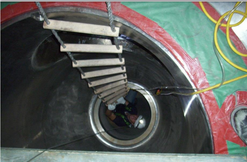
Inspector entering the reactor coolant pump bowl
