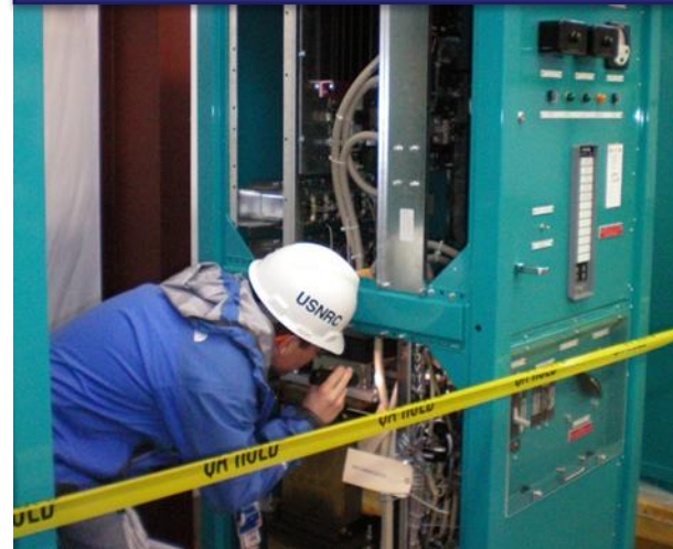
Receipt/Storage inspection of vital inverter
