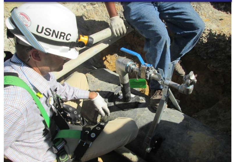
Inspection of vent installation
