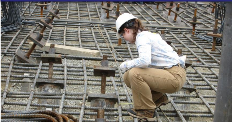
Inspection of rebar placement
