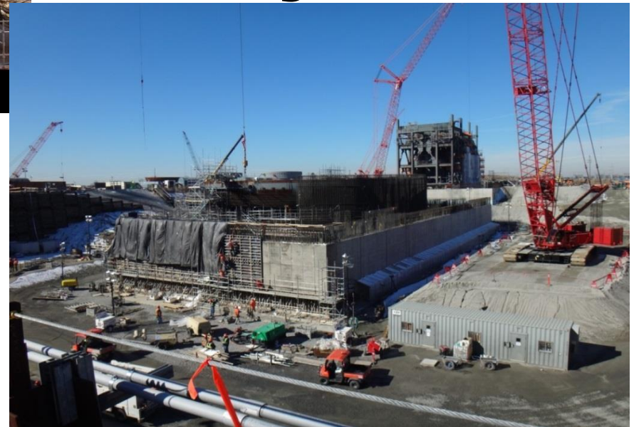
The 1,100-ton CA20 module is placed into Plant Vogtle Unit 3 nuclear island. The module, which is more than five stories tall, will house various plant components, including the used fuel storage area.
