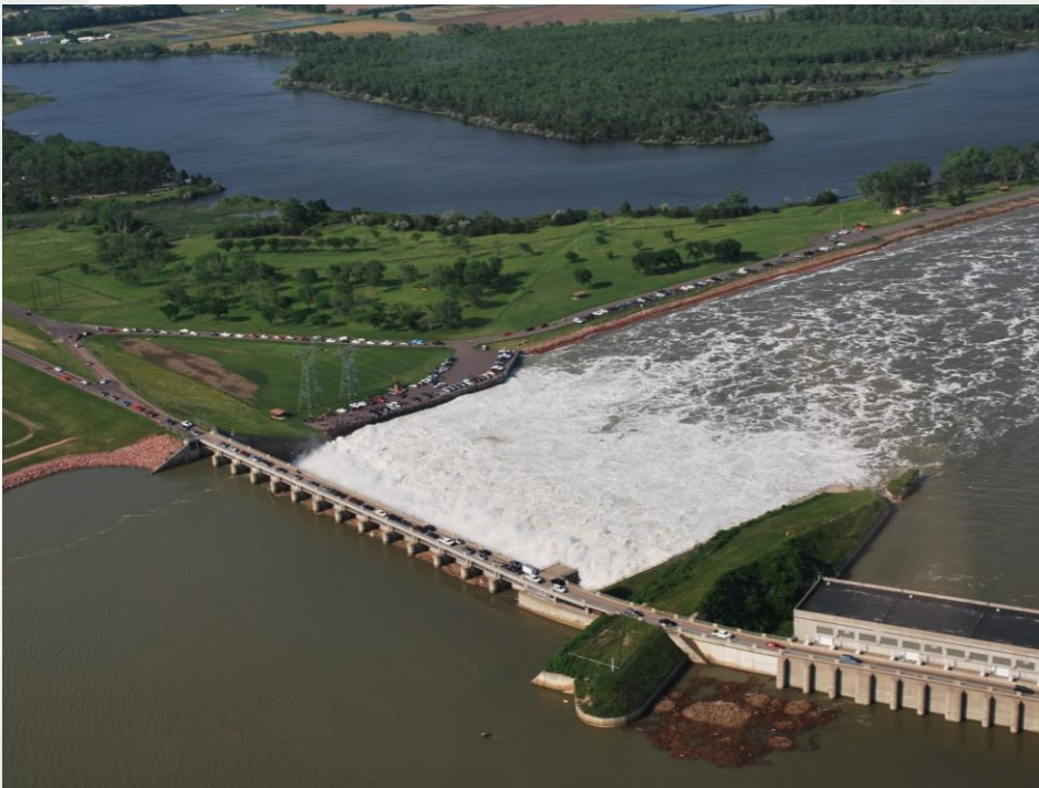
GAVINS POINT DAM
