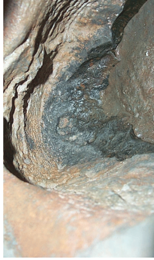
Close-Up View of Cavity
