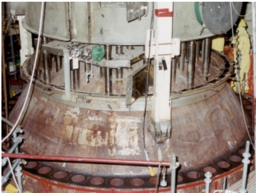
Figure 8 Visual Inspection of Salem 1 Reactor Vessel Head
