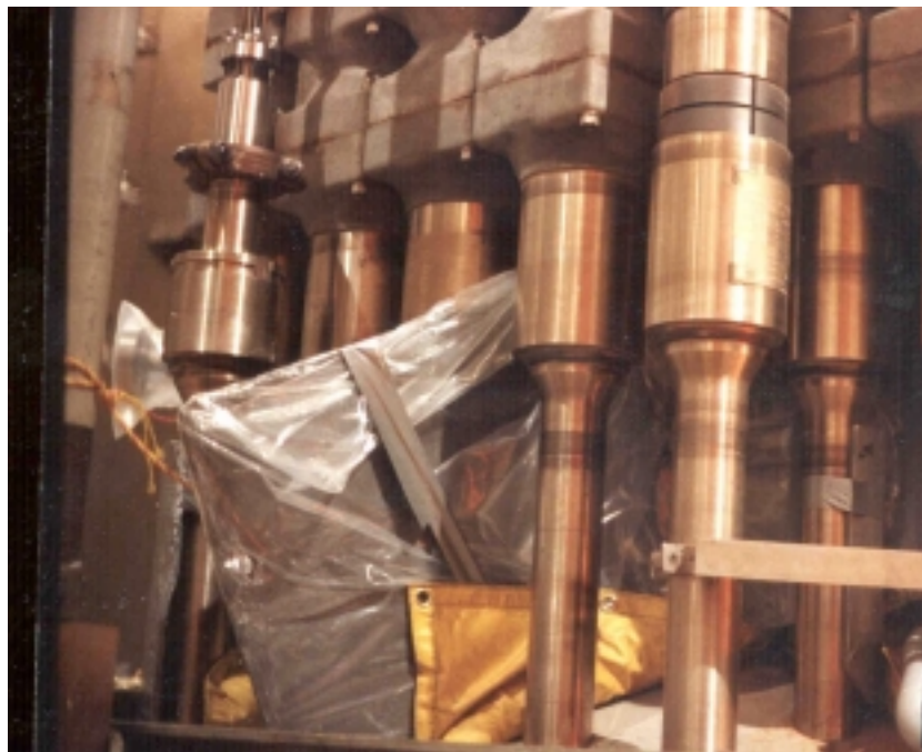
Figure 10 Visual Inspection of Prairie Island 1 Reactor Vessel Head
