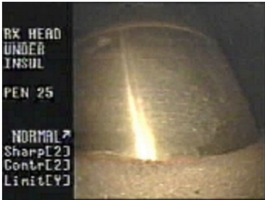
Figure 11 Visual (Video) Inspection of Farley 2 Reactor Vessel Head (Nozzle 25)
