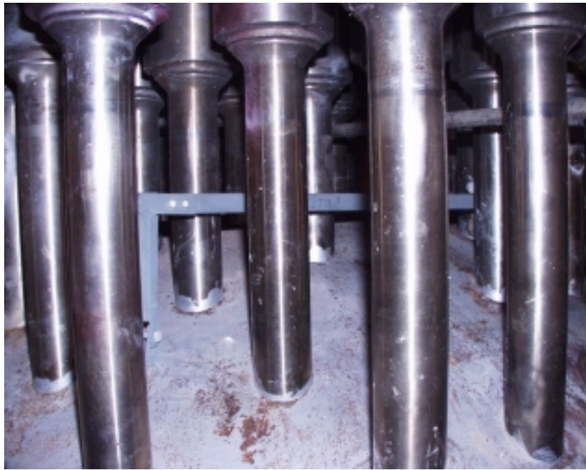
Figure 9 Visual Inspection of H. B. Robinson 2 Reactor Vessel Head
