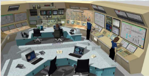
Hybrid Control Room
