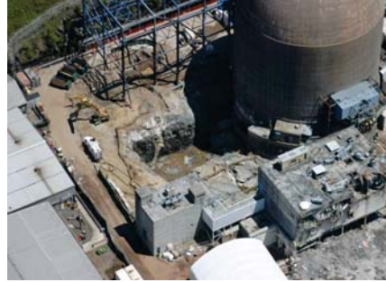
Sr-90 Plume Remediation Area
