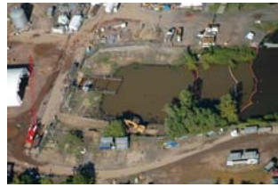
Aerial View of Discharge Canal
