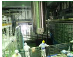
Move of the cask to downstairs
