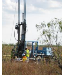
Core Boring starting soon
