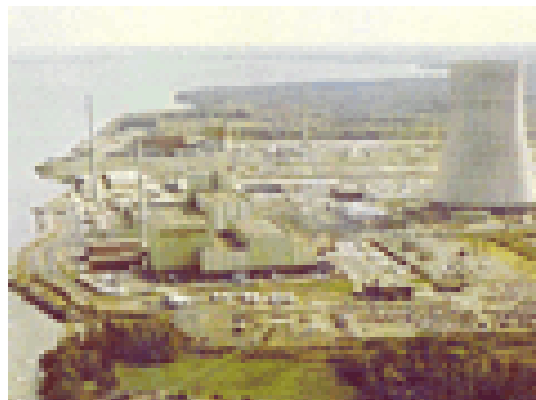
Nine Mile Point, Unit 1
