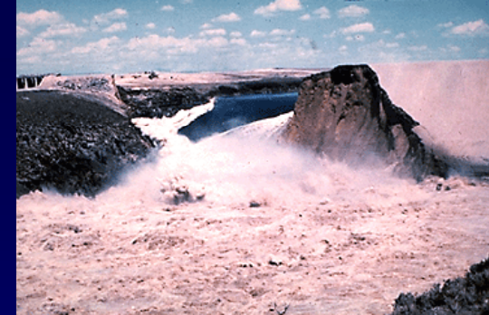
1976 Teton Dam collapse Source: U.S. Bureau of Reclamation
