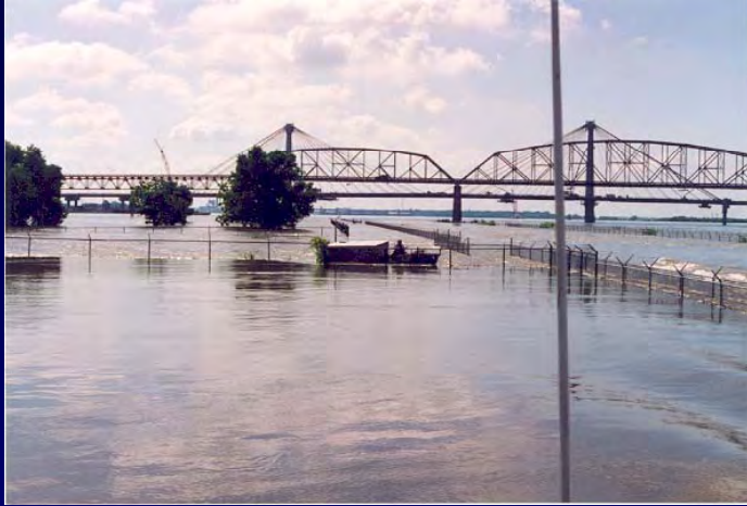
1993 Mississippi River Flooding at Alton IL Source: U.S. Geological Survey
