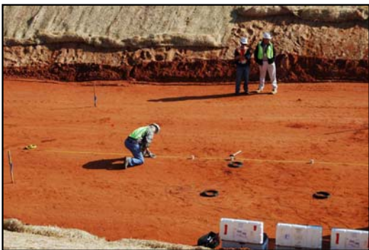
SASW Using Hammer as Source
