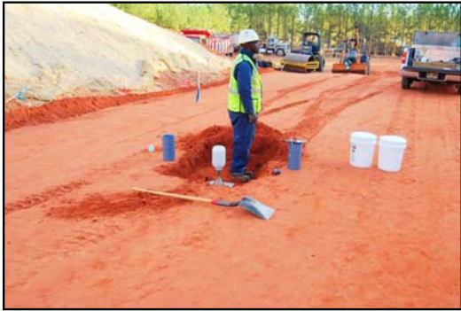
Density Testing Using Sand Cone Method
