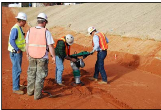
Hand-Compaction after Sand Cone Test
