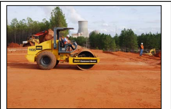
Compaction of Final Layer
