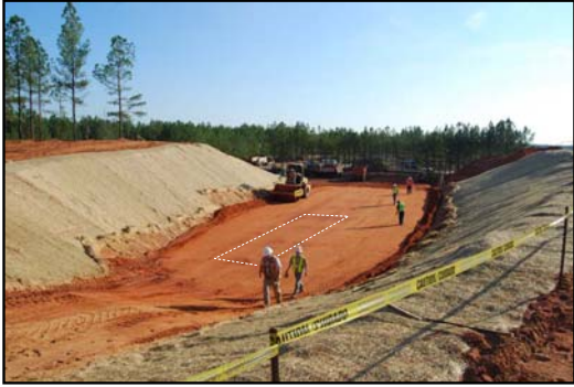
Compaction in Progress
