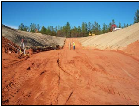
Surveying after Five Feet of Backfill
