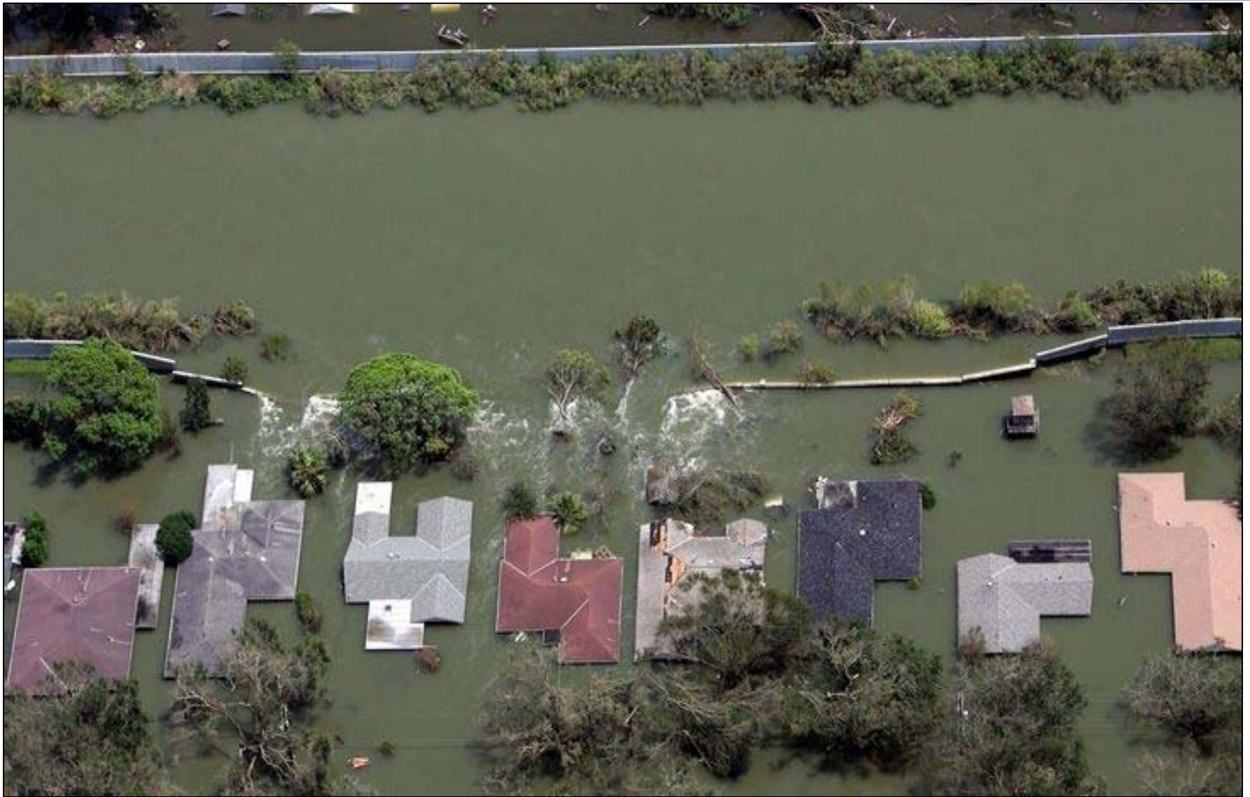
17 th Street Canal
