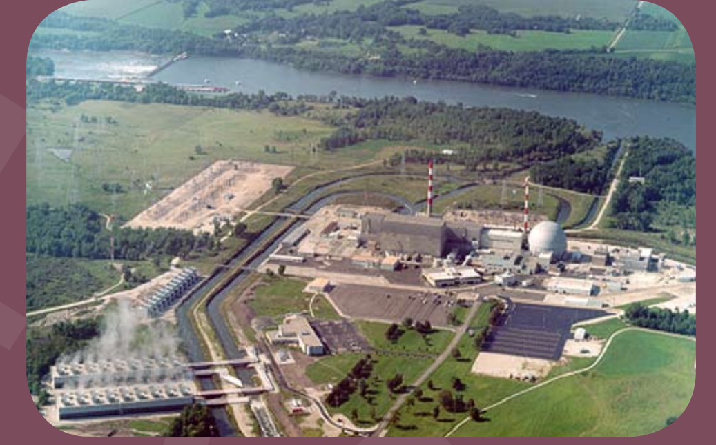
Dresden Nuclear Power Station, Units 2 & 3
