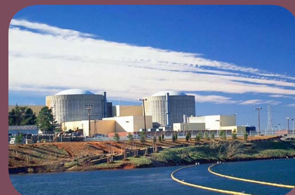
McGuire Nuclear Power Station, Units 1 & 2
