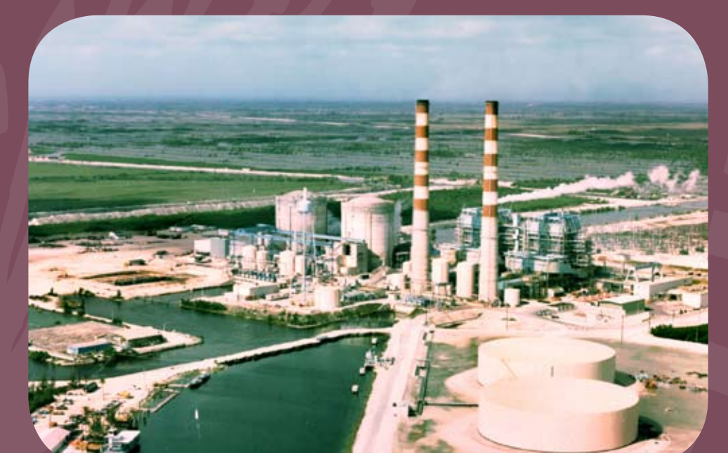
Turkey Point Nuclear Power Plant, Units 1 & 2
