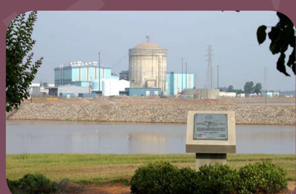
Virgil C. Summer Nuclear Power Station
