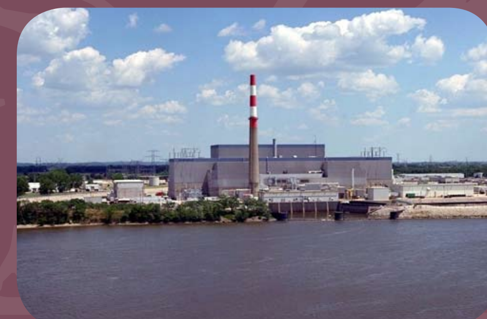
Quad Cities Nuclear Power Station, Units 1 & 2
