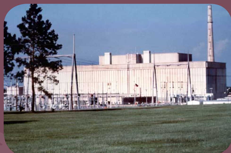
Edwin I Hatch Nuclear Power Plant, Units 1 & 2
