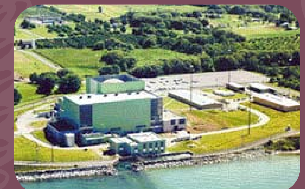
R.E. Ginna Nuclear Power Plant
