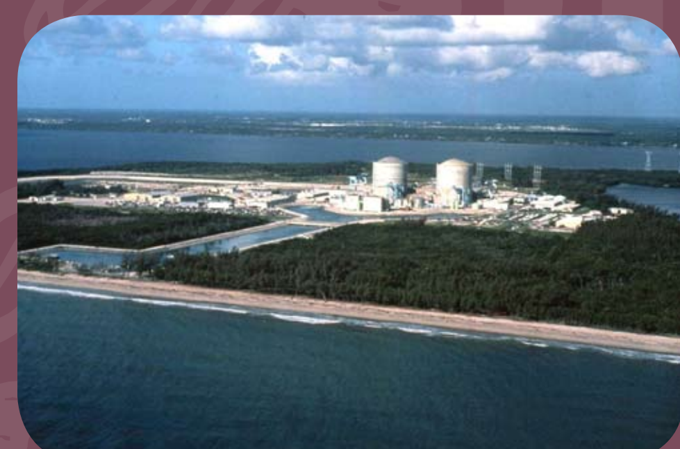
St. Lucie Nuclear Plant, Units 1 and 2
