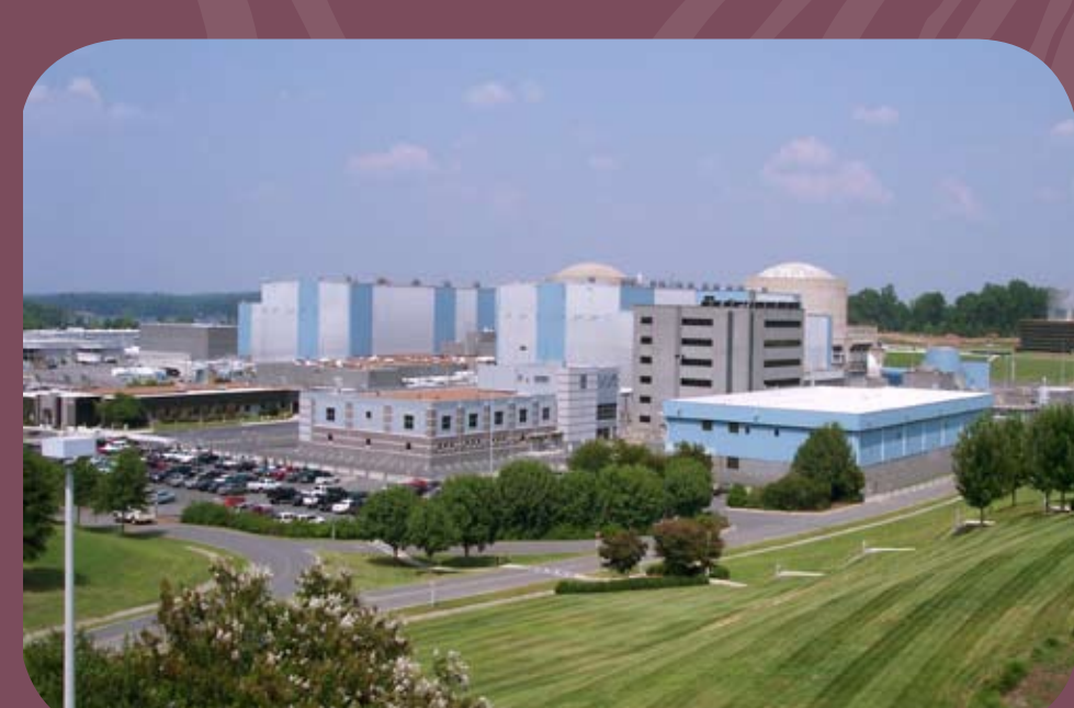
Catawba Nuclear Station, Units 1 & 2
