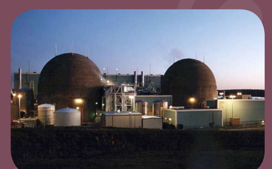
North Ann Power Station, Units 1 & 2
