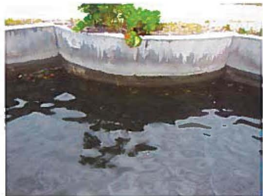
Photo 2-1. Hardened shoreline of barge canal
