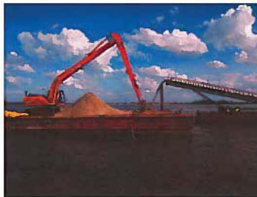
Photo 3-3. Fill conveyor loading placement barge
