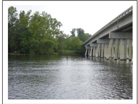
Looking south at study area along bridge.
