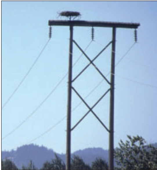
FIGURE 6.22: This osprey nest was originally located on the crossarms above the center conductor where contamination from fallen nest material and excrement accumulated. It was relocated to the platform shown. A halved, corrugated pipe was installed to prevent re-nesting on the crossarms. Relocating a problem nest to a nest platform on an adjacent non-energized pole is preferred. However, if pole cost, rights-of-way restrictions, or limited access prevent installation of a new structure, it is best to install a safe nest platform on the existing structure.
