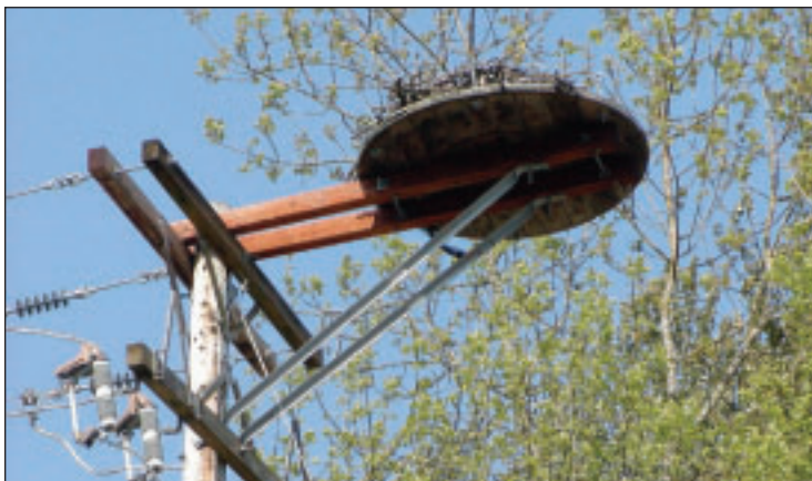
FIGURE 6.10: Osprey nest platform design developed by Portland General Electric. The platform is constructed from the end of a 1.5-meter (m) (5-foot [ft]) diameter wooden cable spool with coated cable along the edge to contain nest material. Utilities should ensure energized parts and equipment below the nest are covered to prevent electrocution of birds or outages from nest material. Consumer's Power, Inc. retrofitted this pole to their avian-safe standards.
