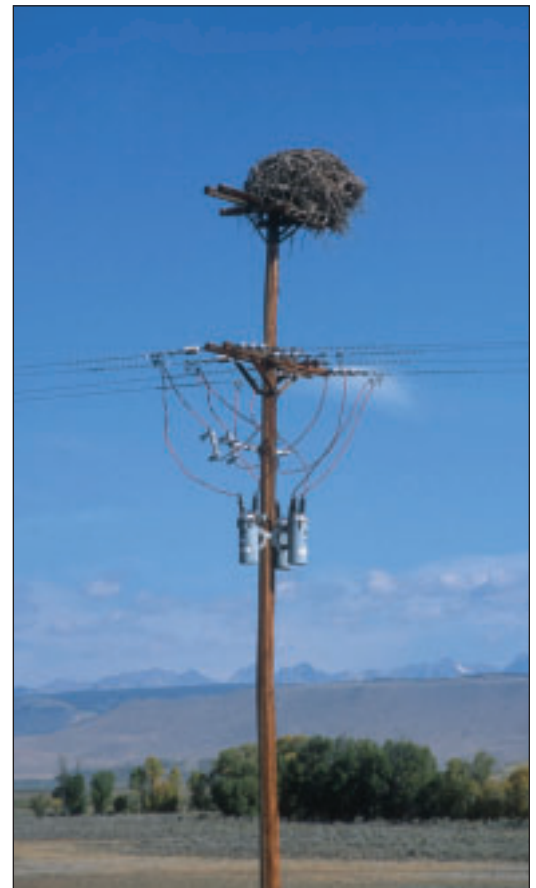
FIGURE 6.16: Osprey nest in Wyoming atop double dead-end pole. Nesting material that may drop onto the conductors or equipment poses fire, outage, and equipment damage risks.
