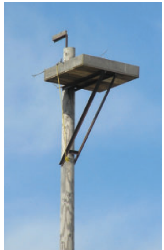
FIGURE 6.14: A simple and cost-effective offset nesting platform built for ospreys in Washington. Pallets can be used as platforms, providing ospreys with a flat nesting area.
