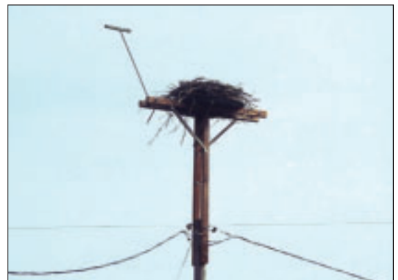
FIGURE 6.11: A nest platform built atop a pole using crossarms to extend the platform above the conductors. This design also includes an optional elevated perch to attract ospreys. The perch should be perpendicular to the prevailing wind.
