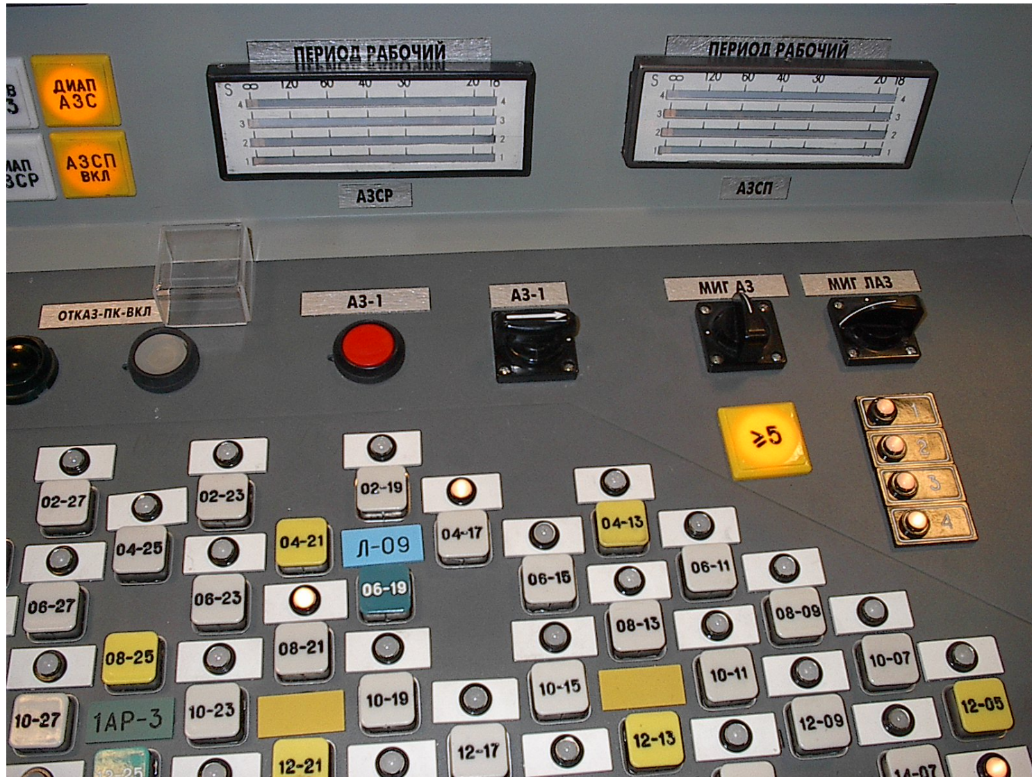
Redundant Reactor Period Meters ( \infty , 10sec) shown on Control Rod Panel 42
