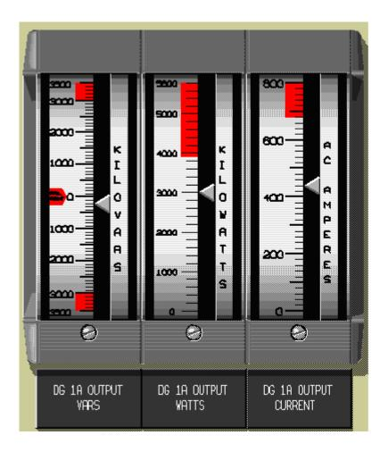
As the 1A DG voltage regulator switch is taken to the "Raise" position, which direction will the needle on each meter INITIALLY move?
