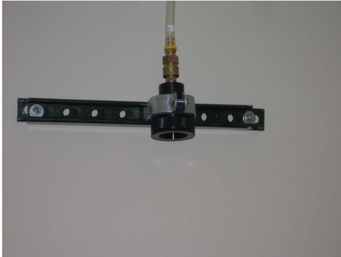
Room air sample head in Iodine room
