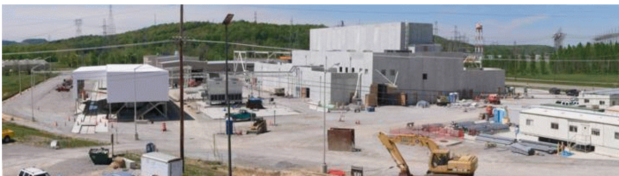
Figure 7-17. Deconversion Facility Under Construction at Portsmouth
