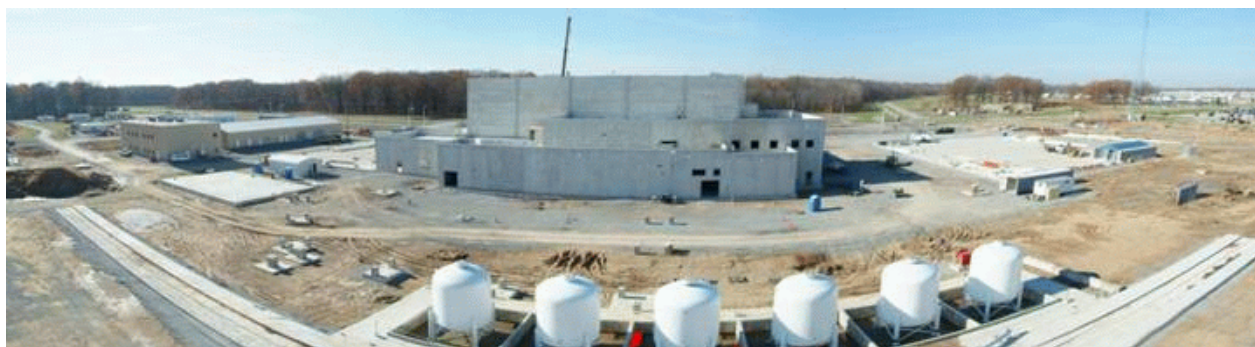
Figure 7-16. Deconversion Facility Under Construction at Paducah
