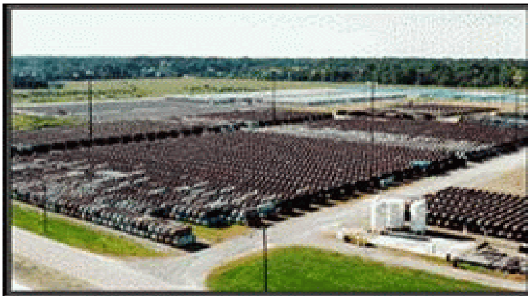
Figure 7-3. Depleted \text{UF}_6 Cylinder Storage Yard at a Gaseous Diffusion Plant Site
