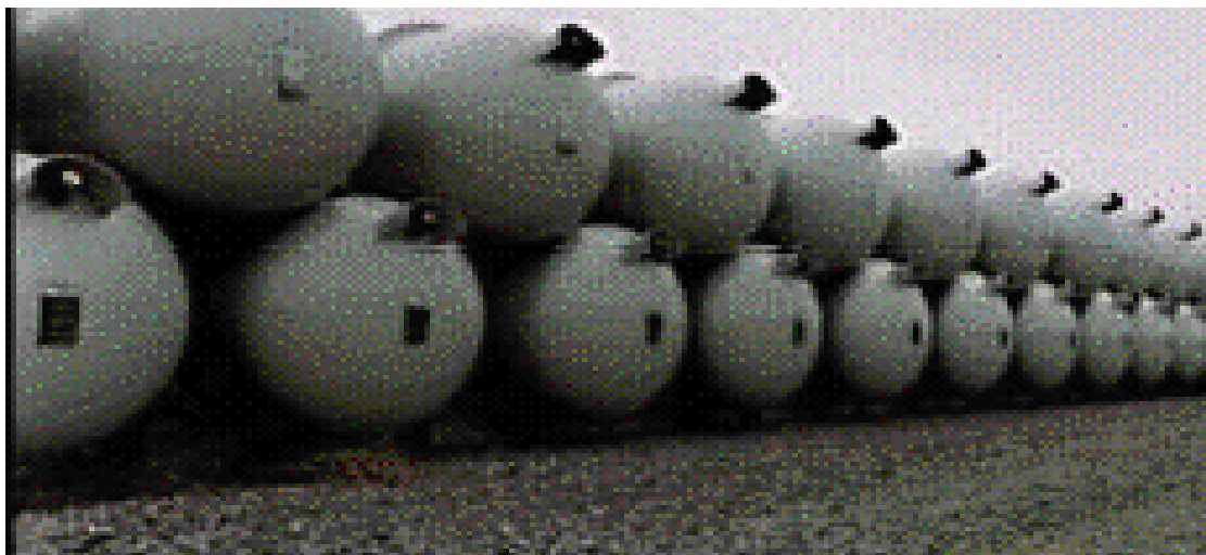
Figure 2-52. Portsmouth Depleted Cylinder Storage Yard. Source: Portsmouth Tour
