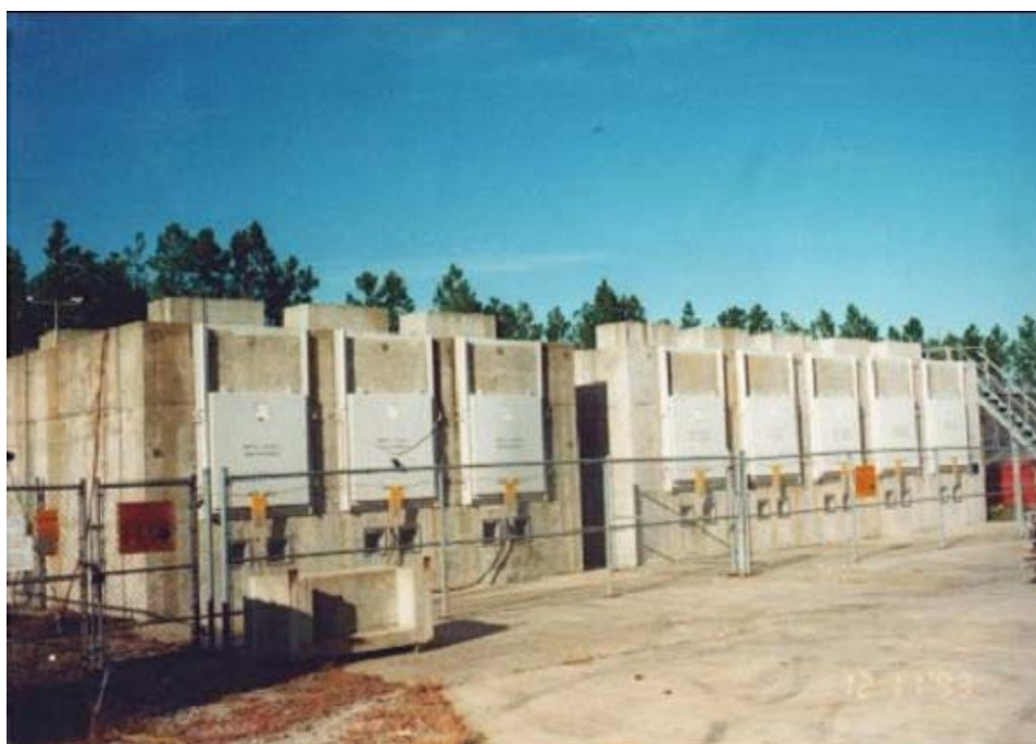
Figure 6-13. Horizontal Modules for Dry Storage of SNF
