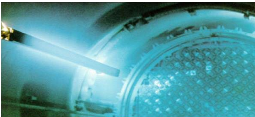
Figure 6-1. SNF Assembly Being Removed During Refueling
