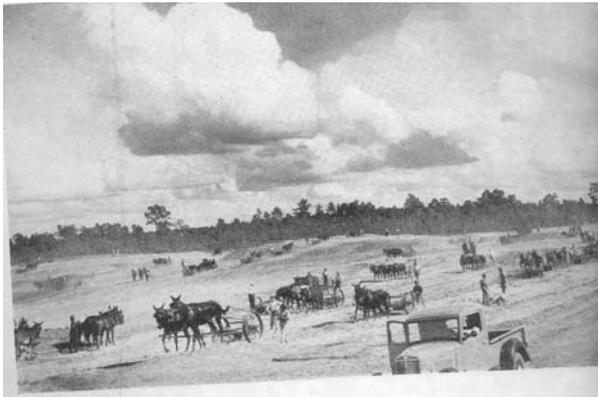
Excavation procedures were a remarkable mix of modern technology and old-fashioned muscle. "Working alongside the modern, powerful excavating machines were men loading trucks with shovels and mule teams dragging old-fashioned scrapers. Huge tractor-scrappers, draglines, belt conveyers, tractor-hauled wagons, and trucks all
