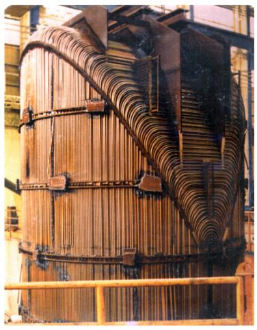
A nuclear steam generator (these are US models, not CANDUS) is an enormous vessel with steel walls. It is a nuclear "boiler". However, the water from the core of the reactor (called the "primary coolant") is not allowed to boil; instead, the primary coolant runs through thousands of small tubes that act as heating elements to boil other water called "secondary coolant". The steam from the secondary coolant is then used to spin a turbine and generate electricity.
