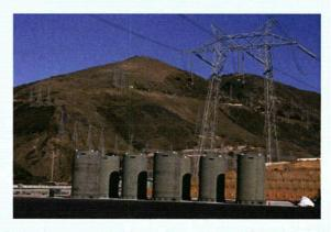
storage overpack that consists of 8 to 10 inches of steel or several feet of concrete (2 to 3 feet). The natural flow of air around the cask in the overpack provides adequate cooling for the spent fuel inside.
