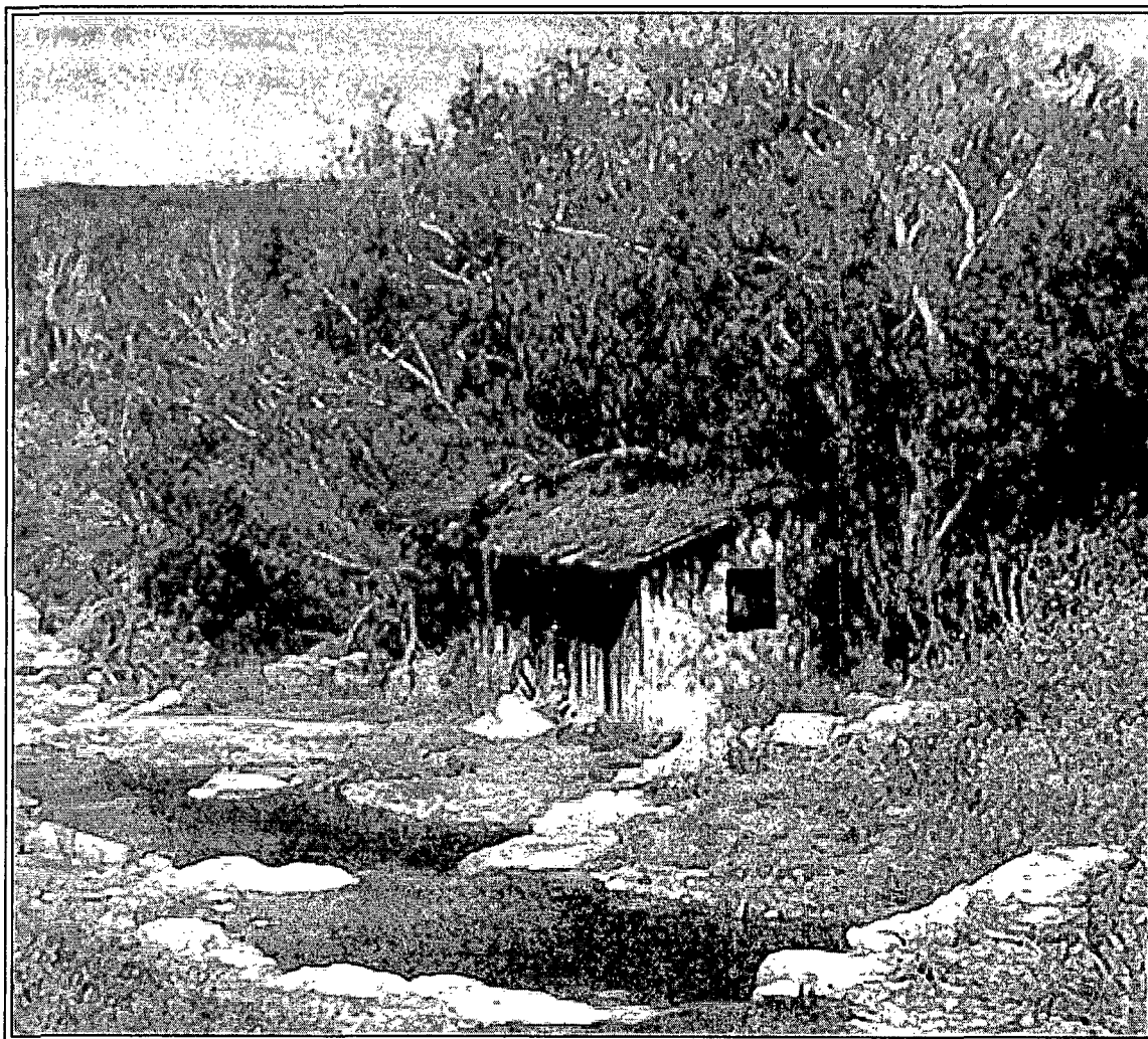
Figure 7.1-1. Historic pump house built in the 1940s, located on Coon Creek within the NRSA.
