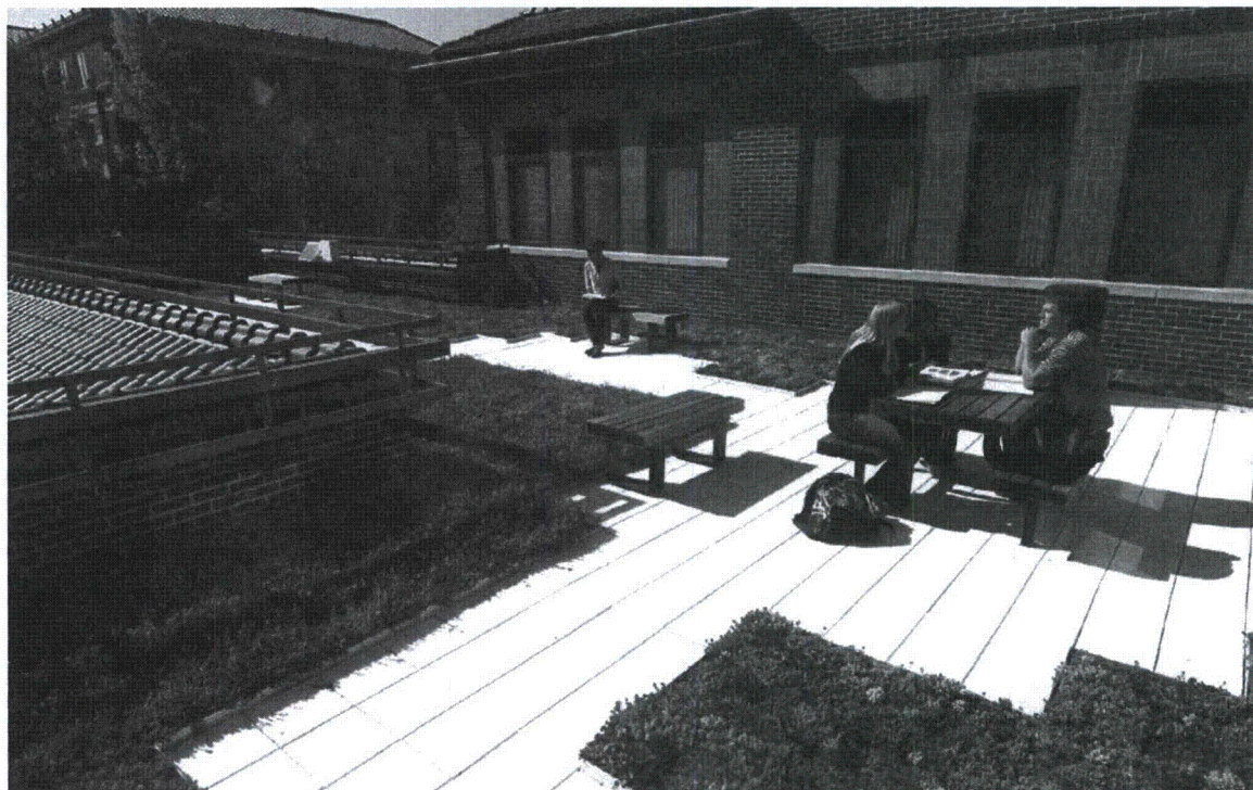
Schleman Hall "green roof"
