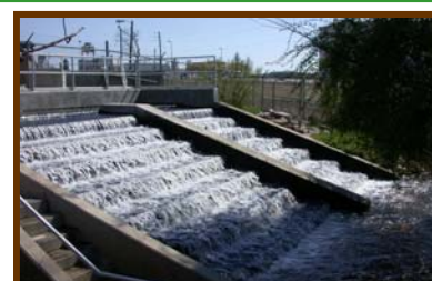
Apex's Water Reclamation Facility final treatment process; cascade aeration
