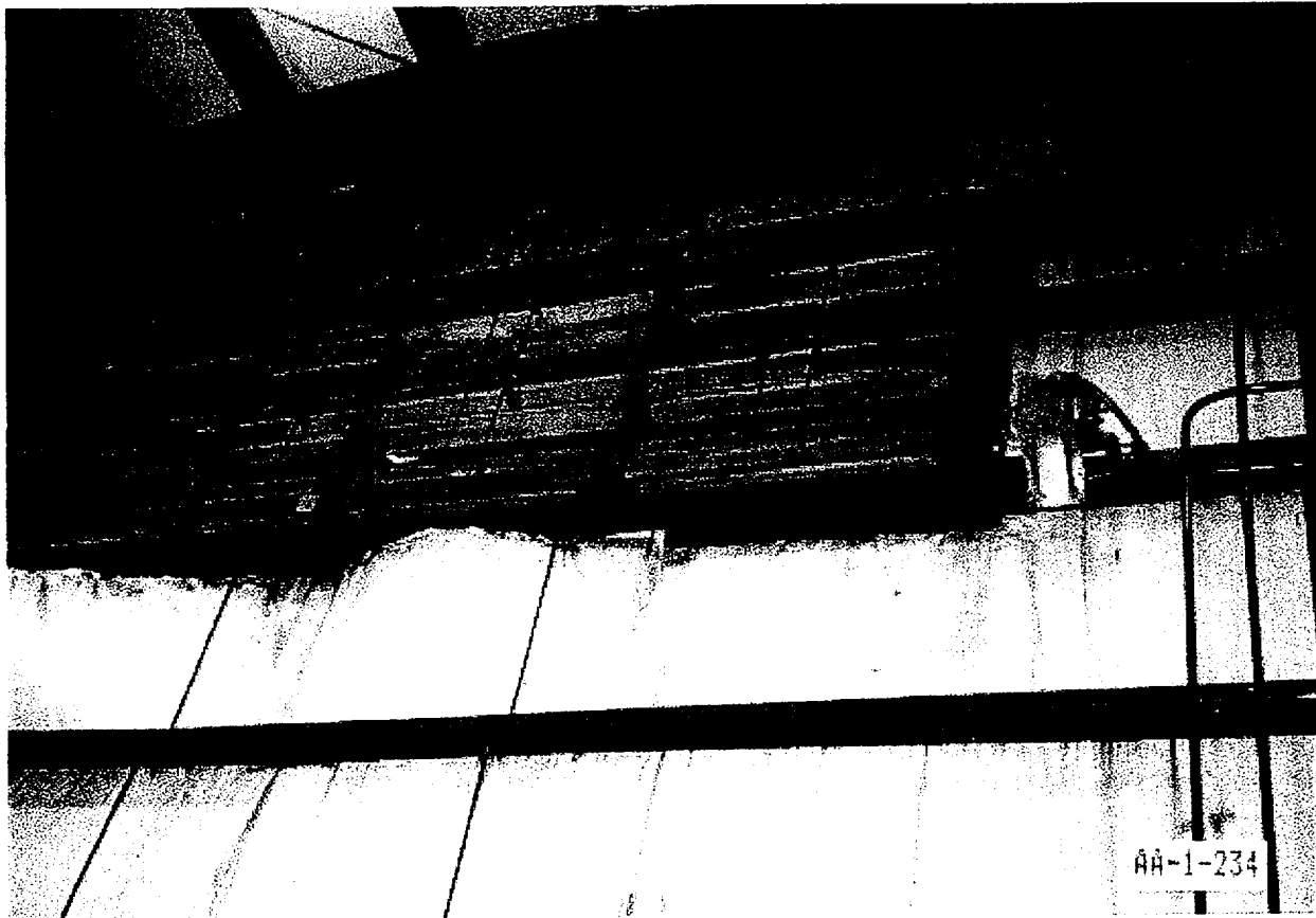
FIGURE A-10: MOTOR-OPERATED DAMPER AT ADAK NAVAL STATION, WHICH EXPERIENCED THE 1986 ADAK ALASKA EARTHQUAKE (0.25G).
