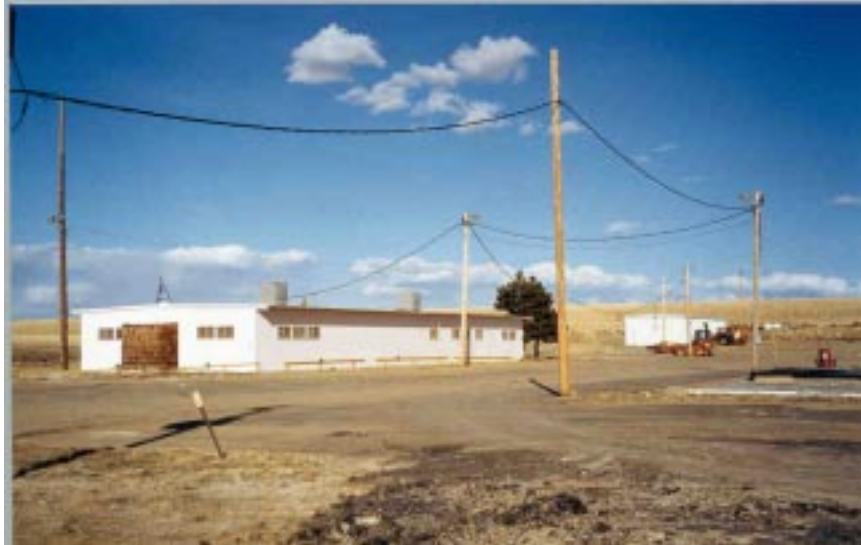
Former site offices scheduled for demolition.
