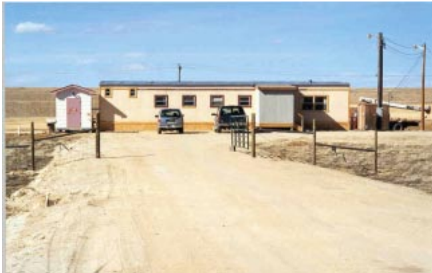
Petrotoomics-Shirley Basin's new site offices.
