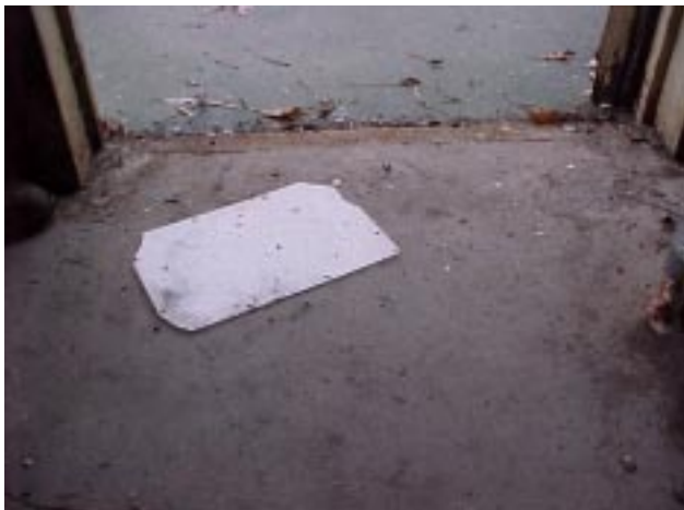
Figure 7 - Cover of Broken Sign (in location where sign was damaged)
