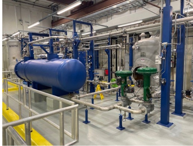
Duke Maintenance Facility
