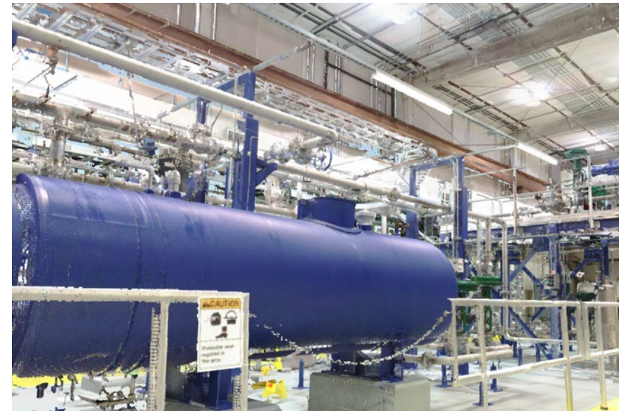
Maintenance Facility Registered Cloudpoint
