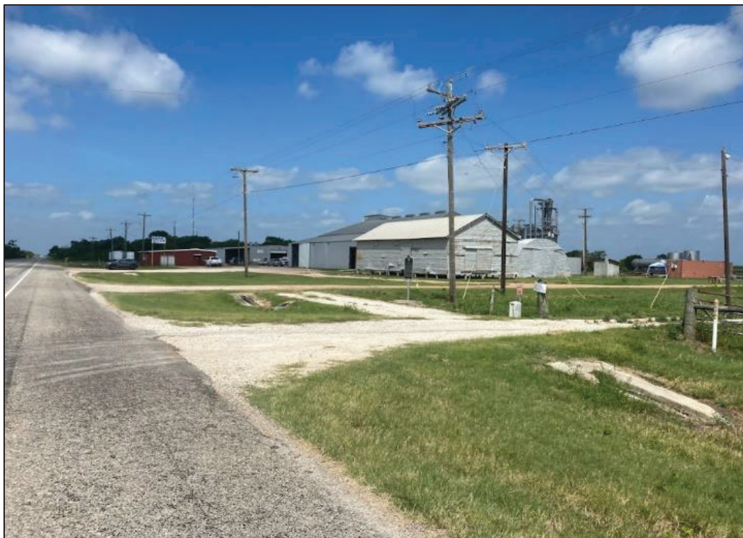
Figure 16.3. Overview of AR 10, facing Northwest.
