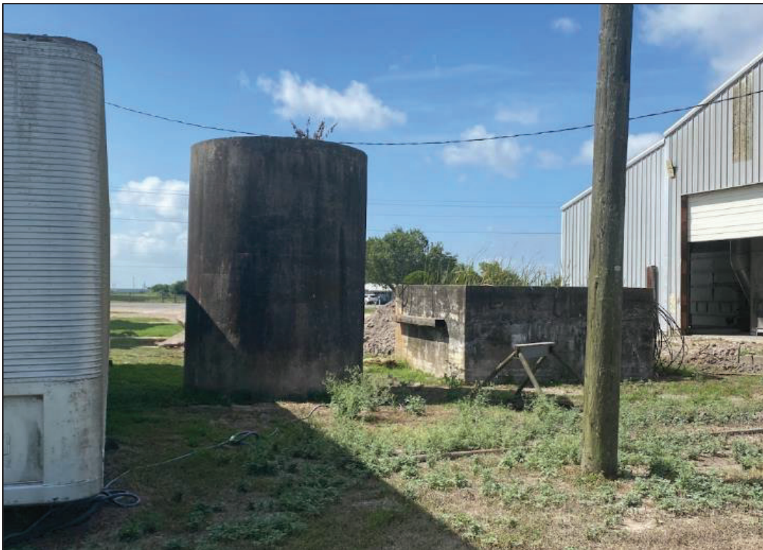
Figure 16.9. View of Earlier Complex Remnants, facing Southwest.
