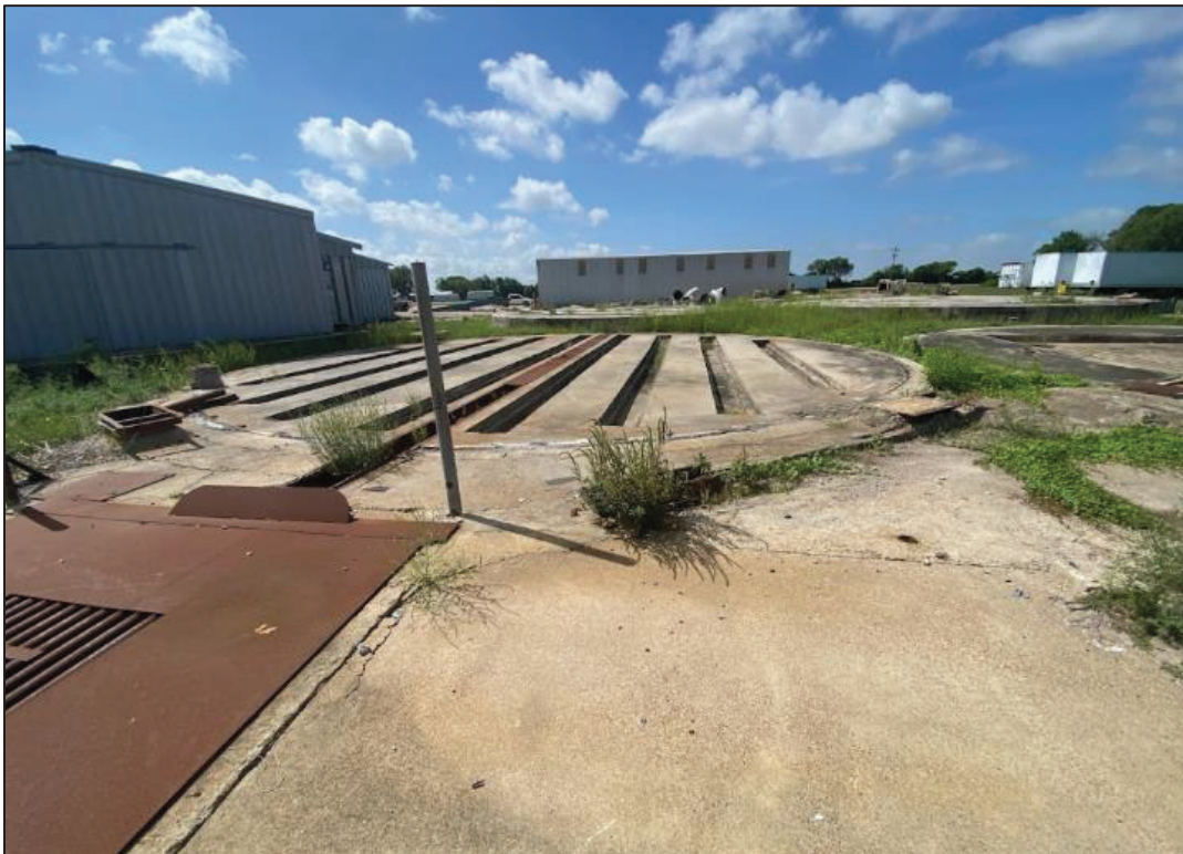
Figure 16.11. View of Grain Bin Foundations, facing South.
