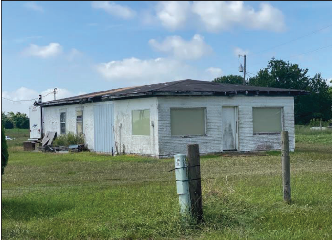
Figure 2.7. Abandoned Residential Structure (AR 9) within the APE.
