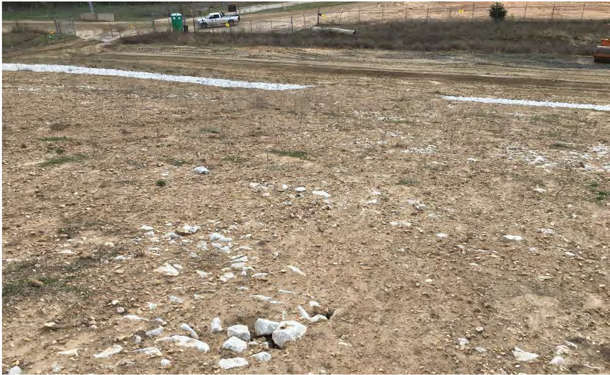
Photo 18. Typical rock mulch surface prior to establishing vegetation, looking down slope to apron bench on east side of Cell (Mar 2021)
