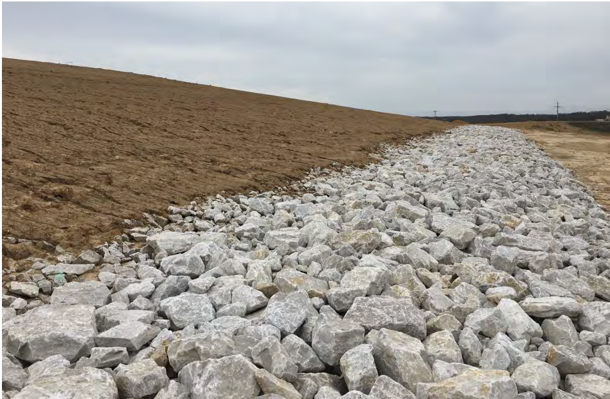
Photo 19. North side of Cell showing apron bench and topsoil-covered slope, looking west (Mar 2022)
