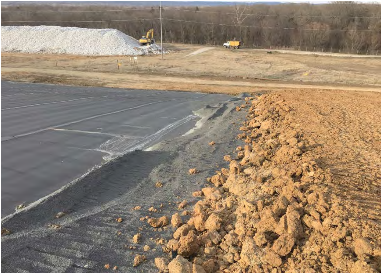
Photo 6. Drainage layer sand and first lift of subsoil placed on cover geomembrane on north side of cell, looking north toward riprap stockpile (Jan 2020)
