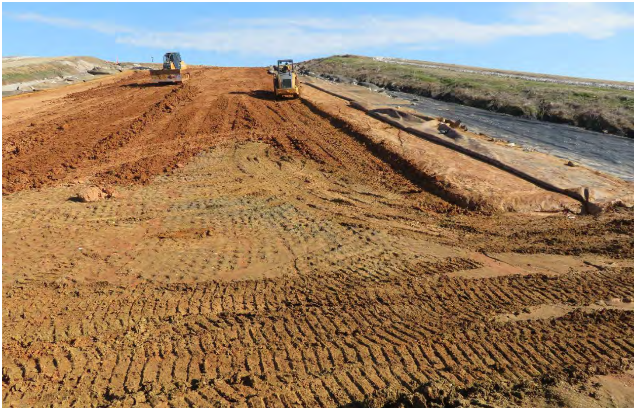
Photo 29. Clay placement and compaction for cover completion in access ramp on south side of Cell (Feb 2025)
