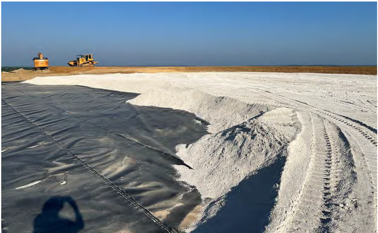
Photo 21. Cover geomembrane, drainage sand, and subsoil on top surface of Cell, looking north (Sep 2023)
