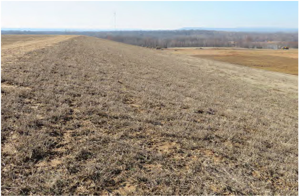
Photo 30. West side of Cell, looking south (Feb 2025)
