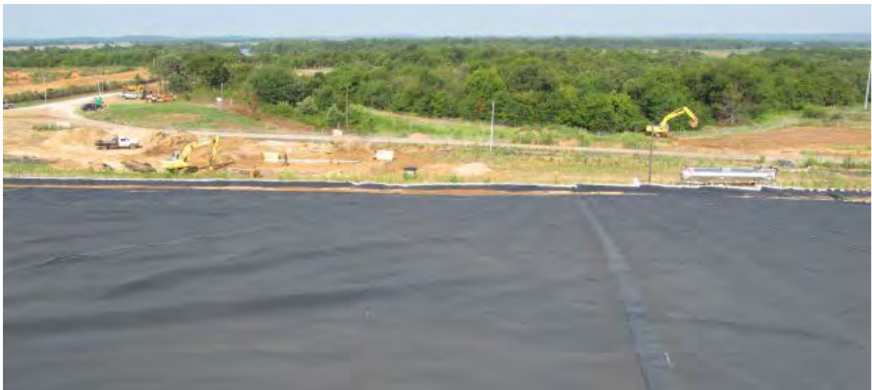
Photo 3. Cover geomembrane on west side of Cell, looking west (Jul 2016)
