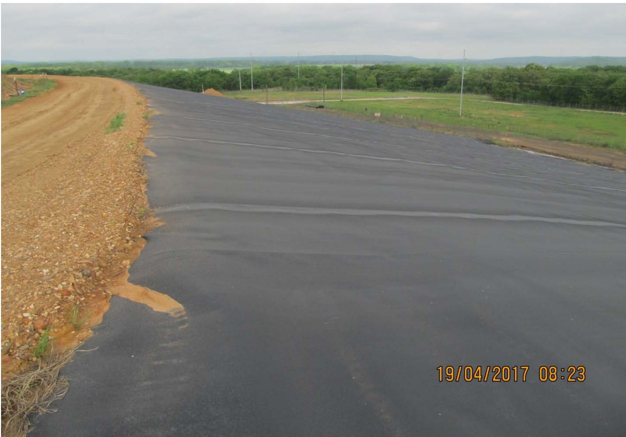
Photo 5. Cover geomembrane on north side of Cell with temporary anchor trench, looking west
