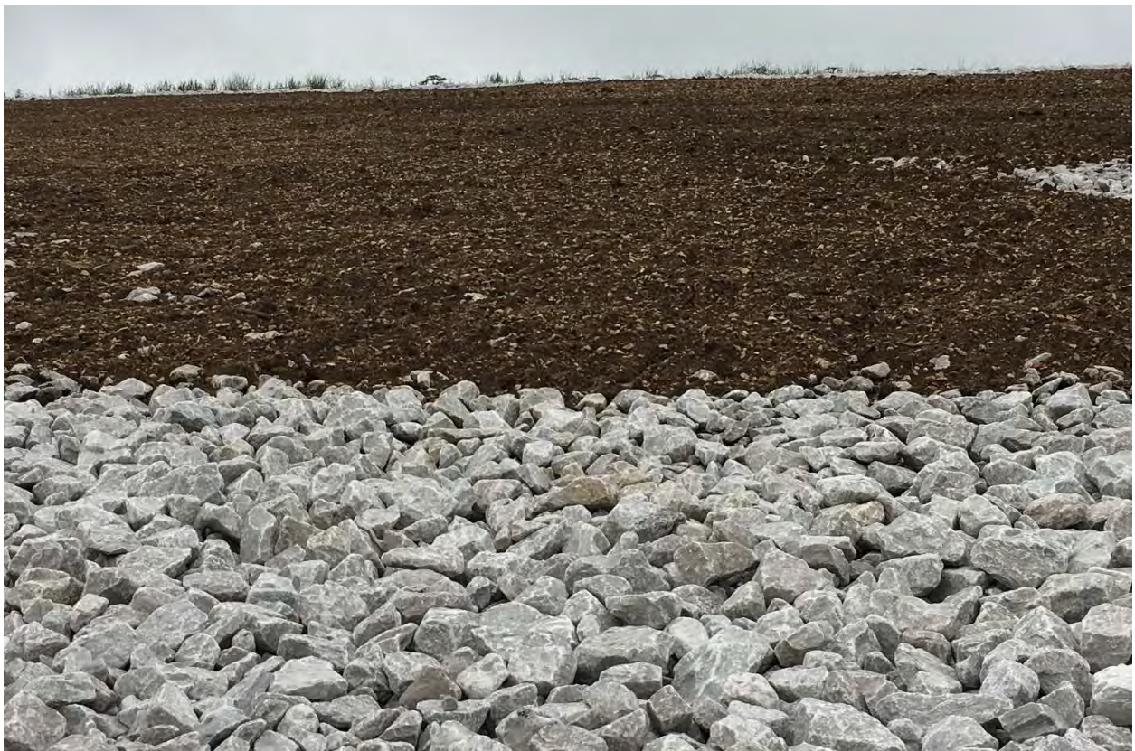
Photo 17. Topsoil spread on top of riprap, looking up slope (May 2020)
