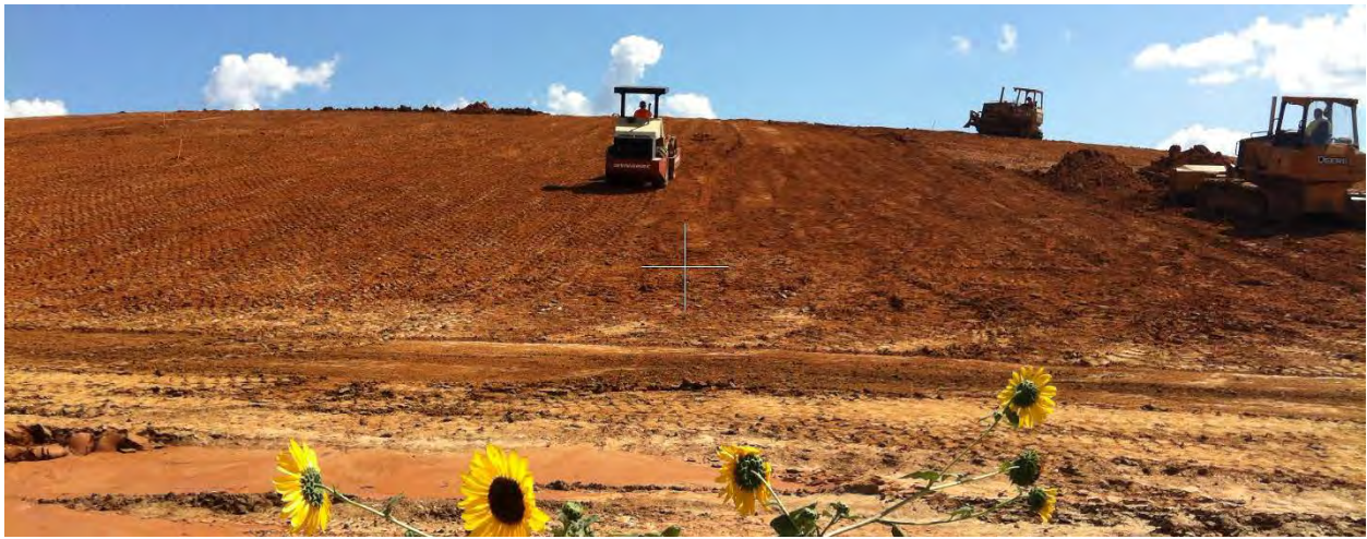
Photo 1. Cover clay liner placement and compaction (Sep 2015)
