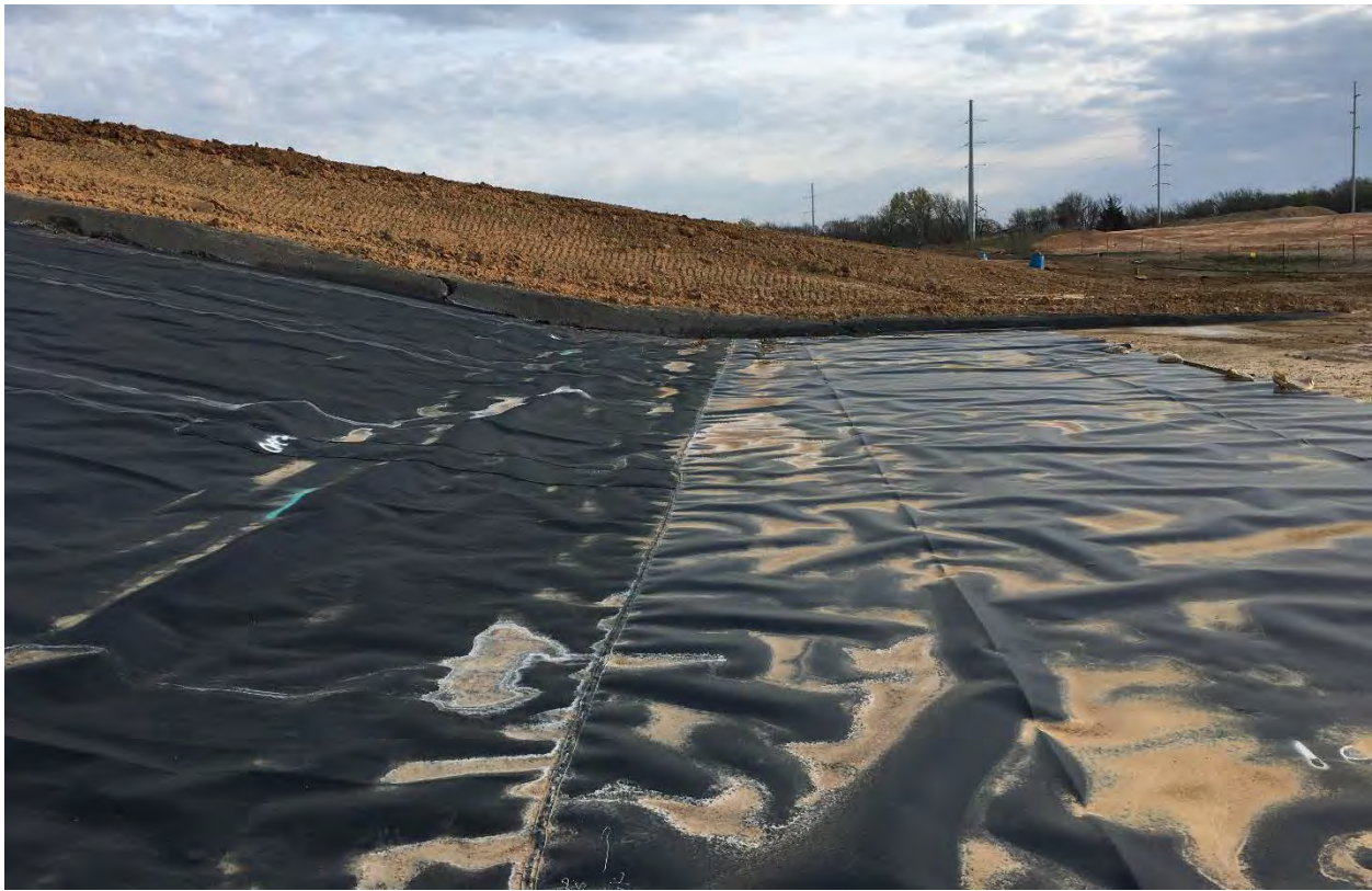
Photo 8. West side of Cell showing drainage sand and multiple lifts of subsoil on cover geomembrane, looking south (Mar 2021)
