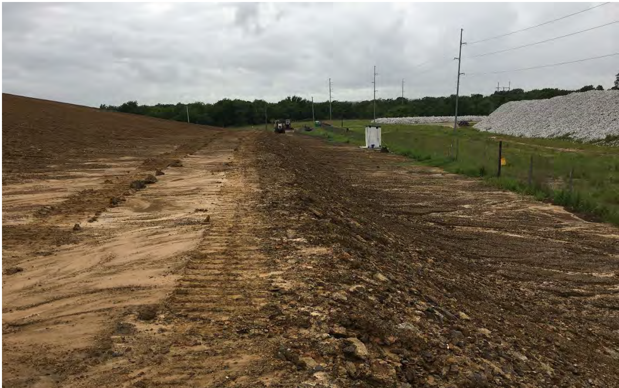
Photo 10. Apron bench on north side of Cell prior to apron rock and slope riprap placement, looking west (May 2020)
