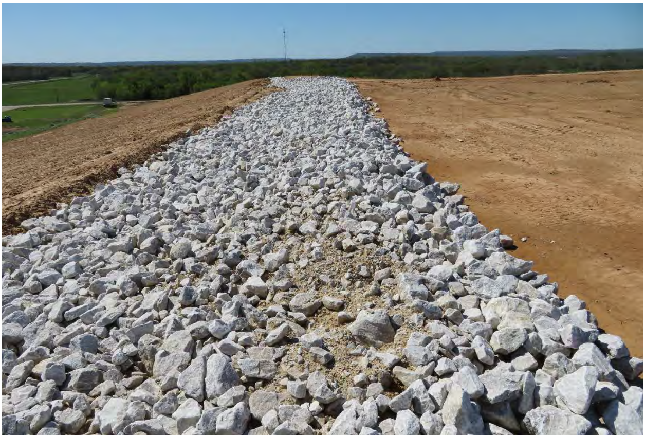
Photo 27. Extension of riprap onto top surface of Cell, prior to covering with topsoil, looking south (Apr 2024)
