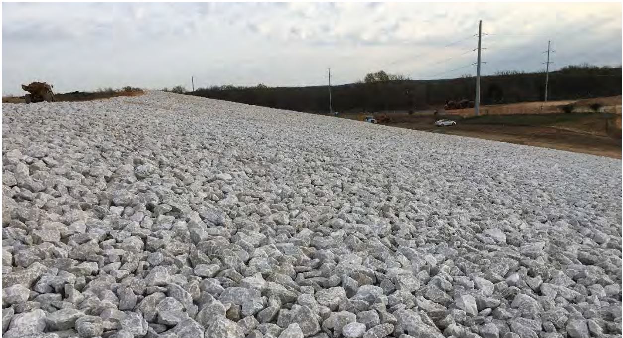
Photo 16. East side of Cell, showing riprapped surface, looking north (May 2020)
