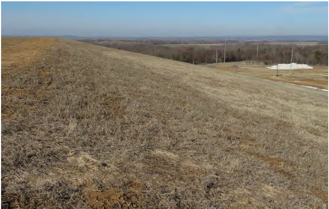
Photo 31. North side of Cell, looking west (Feb 2025)
