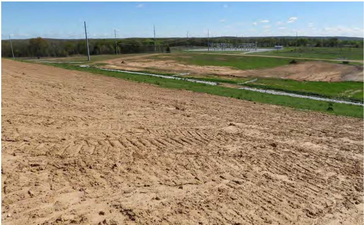
Photo 25. Topsoil-covered riprap on upper surface of east side of Cell, looking northeast over East Diversion Channel and new OG&E substation (Apr 2024)
