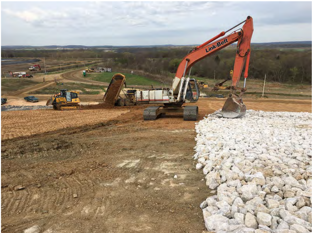
Photo 15. West side of Cell, showing subsoil and riprap placement, looking west (Mar 2021)
