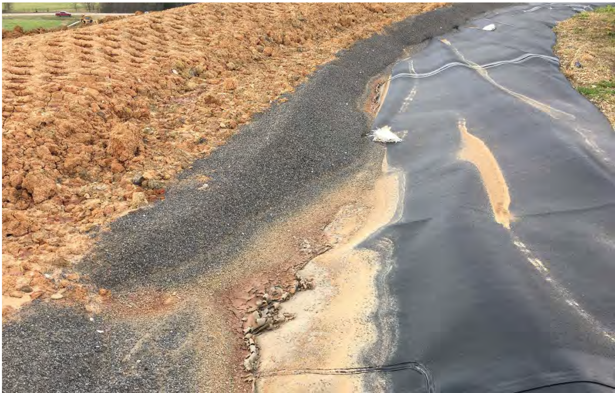
Photo 11. Extent of cover layers on east side of Cell, showing subsoil, drainage sand, and geomembrane in temporary anchor trench, looking south (Mar 2021)
