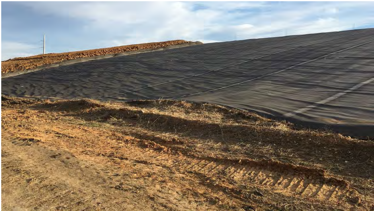
Photo 7. North side of Cell showing initial lifts of drainage sand and subsoil on cover geomembrane, looking southeast (Jan 2020)
