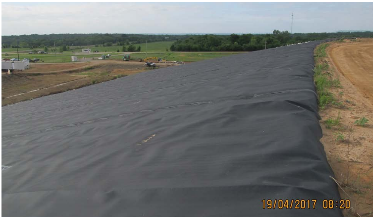
Photo 4. Cover geomembrane on east side of Cell with temporary anchor trench, looking south
