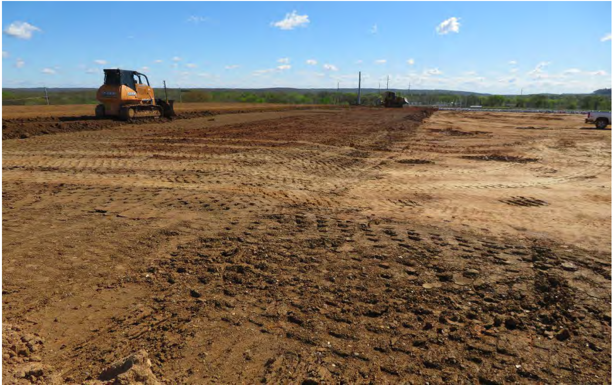
Photo 24. Topsoil placement on top surface of cell, looking east (Apr 2024)
