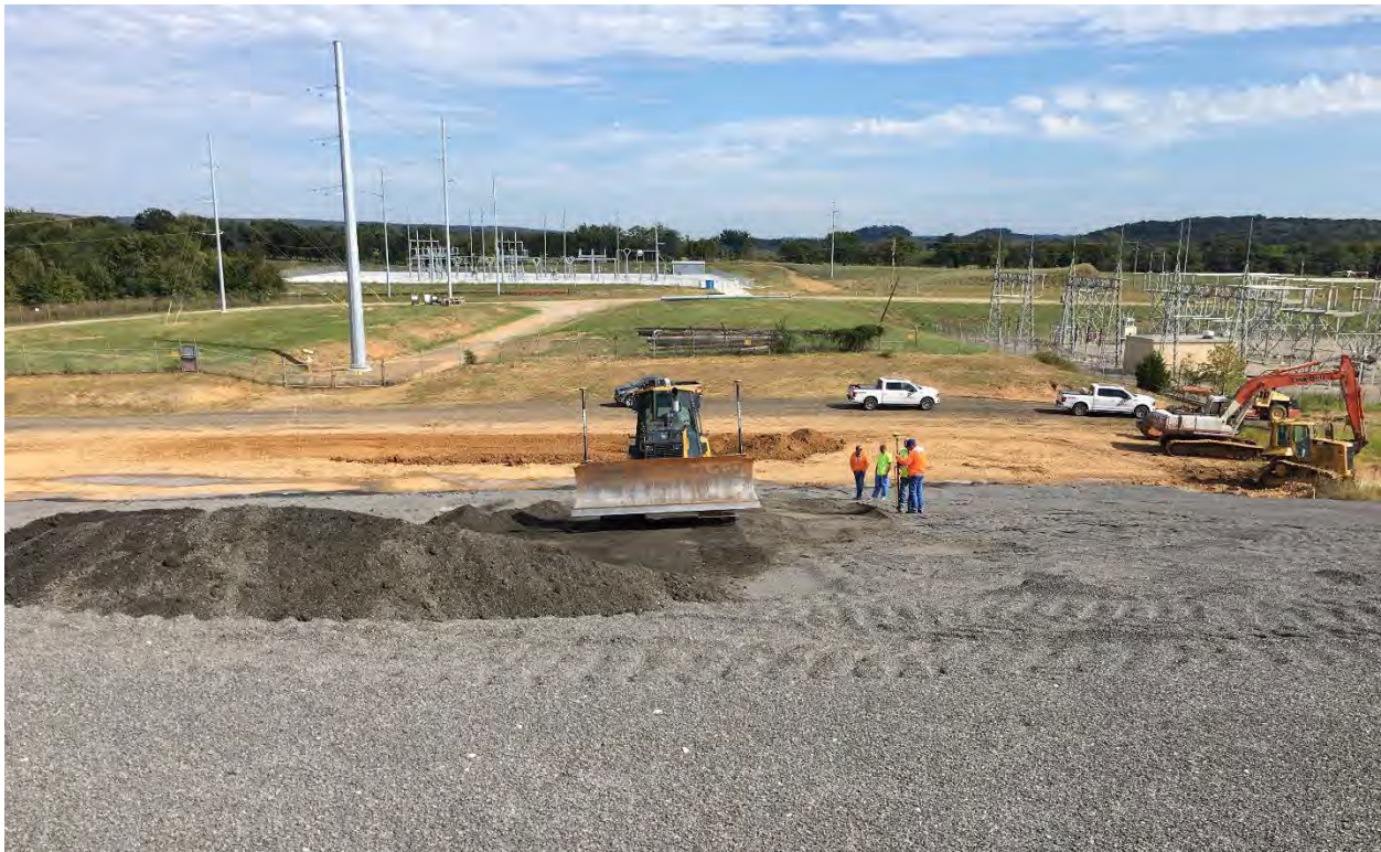
Photo 9. East side of Cell showing drainage sand placement on geomembrane, with former and new OG&E substations in the background, looking east (Oct 2019)
