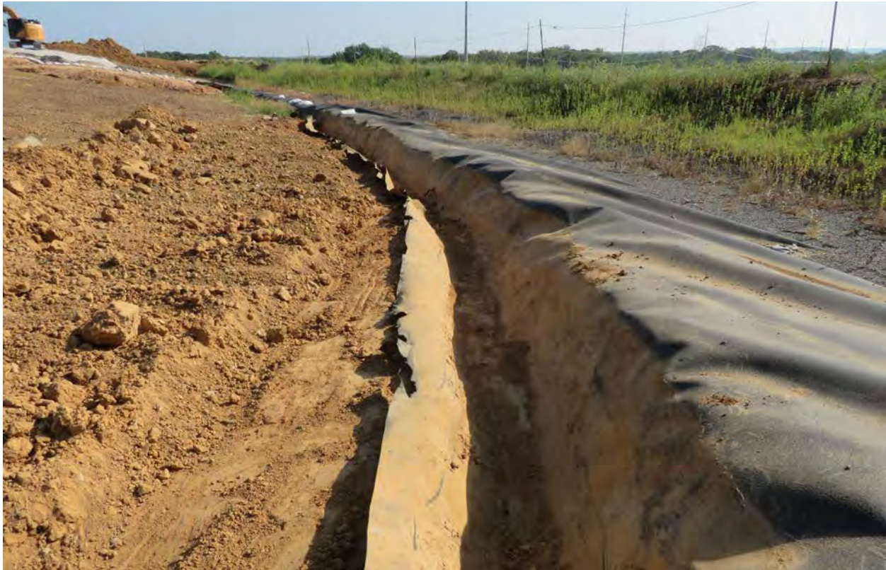
Photo 12. Cover geomembrane on east side of Cell, removed from temporary anchor trench in preparation for extension of cover system to top of cell, looking north (Sep 2023)
