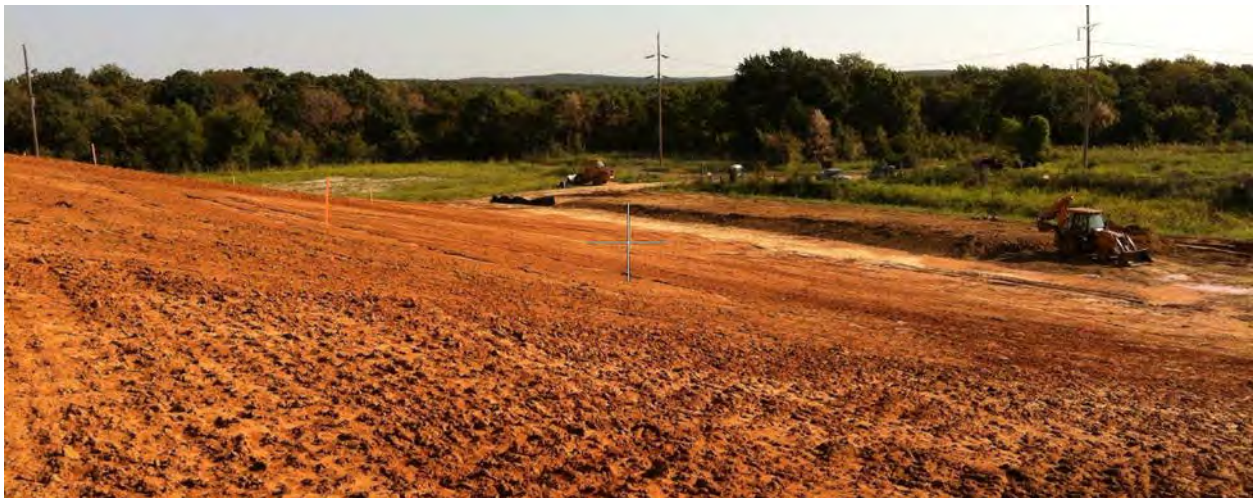
Photo 2. Cover clay liner on east side of Cell, looking northeast (Sep 2015)
