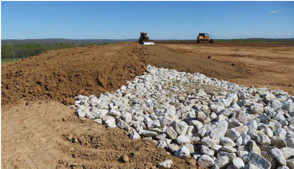
Photo 28. Placement of topsoil over the extension of riprap onto top surface, west side of Cell, looking north (Apr 2024)
