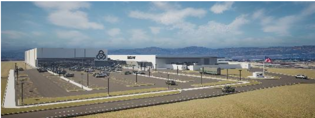
Radiant's full scale manufacturing site at the same Oak Ridge, TN campus.
