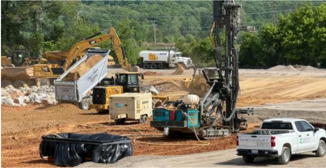
Construction of Radiant's Oak Ridge, TN facility is underway, 6 days/week.
