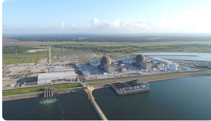
South Texas Project (STP)
