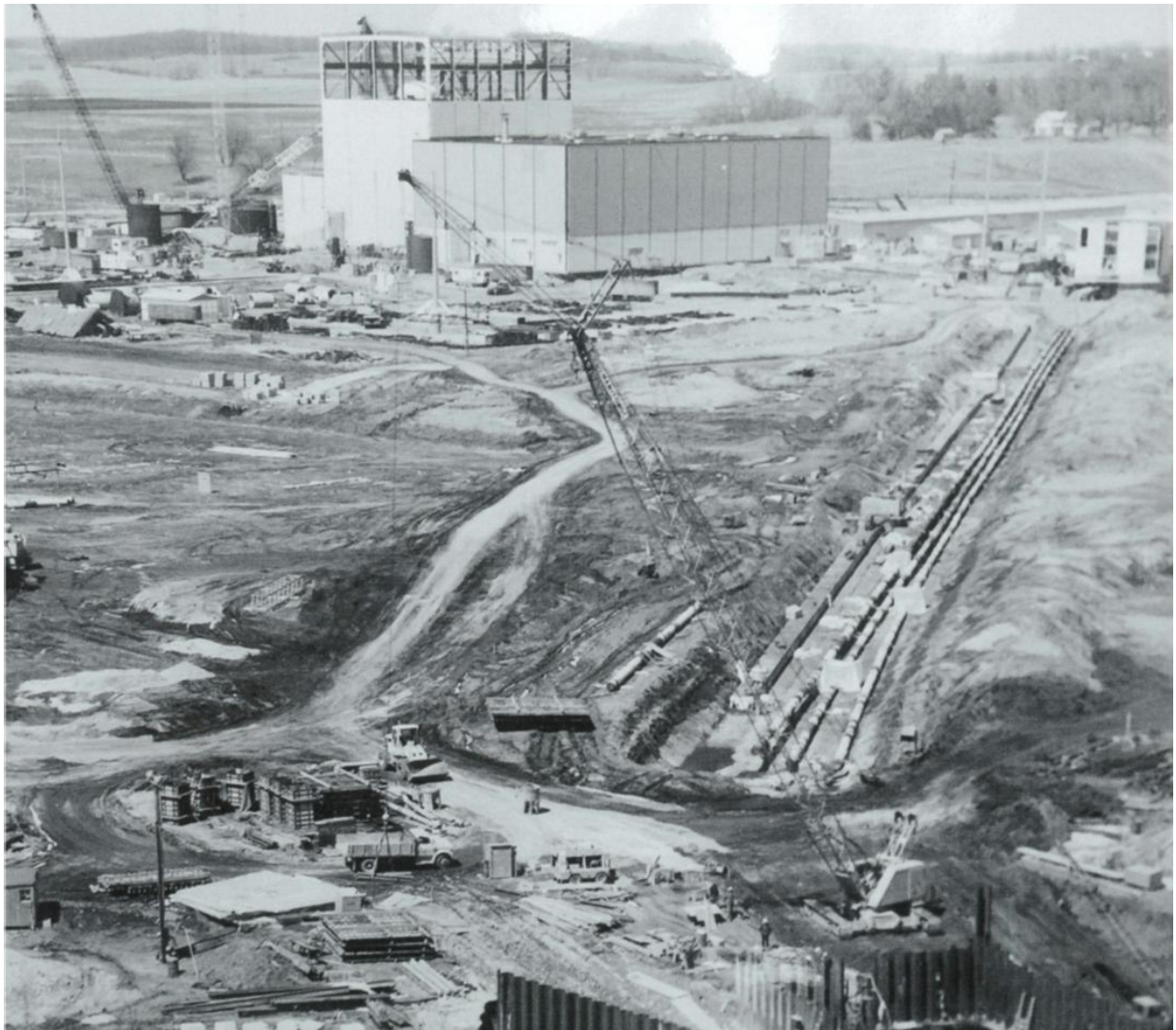
1 2 Figure E-2 The Duane Arnold Energy Center Site During Construction, 1970–1974. View 3 Looking Approximately Northwest. Source: NextEra 2020-TN13420.
