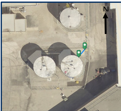
2/3 Condensate Storage Tanks
