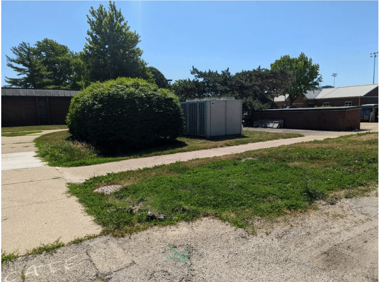
Figure 4-5 View to The Southeast From The Site
