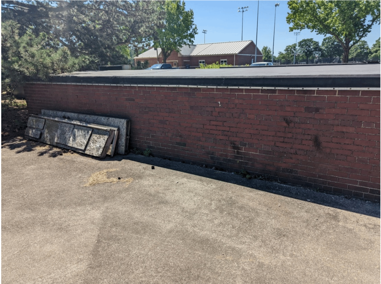
Figure 4-8 GSL Storage Area Located East of The GSL
